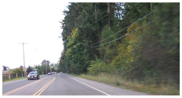
The following photo shows a low make-ready pole line that has only one existing attachment in the communications space. Where make-ready is low, the cost of aerial construction is cheaper than in high make-ready areas.
