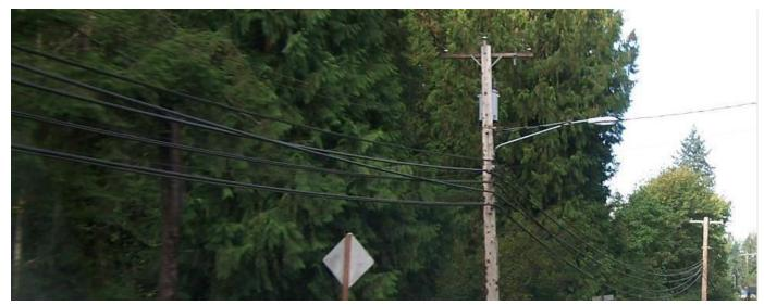
Tree trimming is required to attach an additional attachment on the utility poles in the following picture. Tree trimming is also an important maintenance function necessary to keep the pole line clear of tree limbs that could break and damage the wires on a utility pole.
