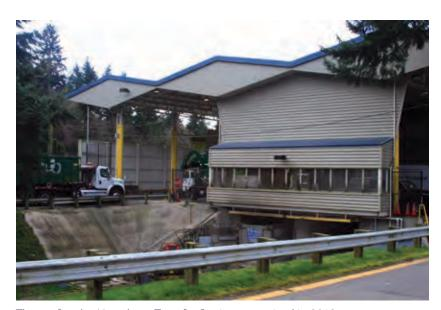
The roof at the Houghton Transfer Station was raised in 2012 to accommodate larger trucks
