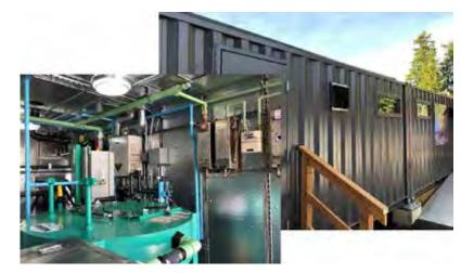
Example of a small anaerobic digester in Redmond (Photo courtesy of Impact BioEnergy, Inc.)
