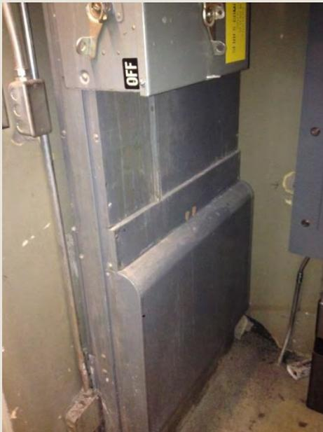
**Figure 1 4000 amp buss electrical buss duct (East Riser)**
