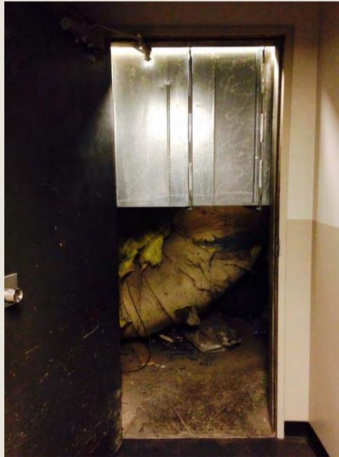
**Figure 2 Access to floor 1A east electrical room by crawling under ductwork, a serious safety hazard and code violation**
