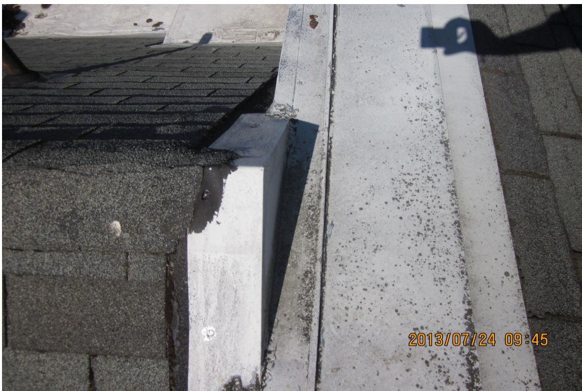
Photo 19. ACM black tar sealant patch on peaked roof.
