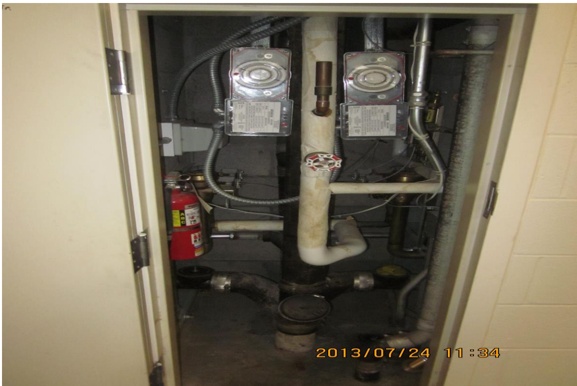
Photo 11. Fiberglass pipe insulation with PVC fittings found throughout Spruce Wing.
