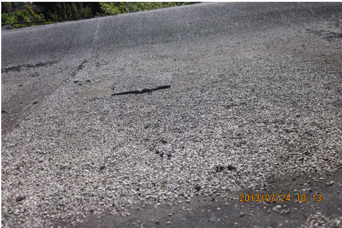
Photo 18. Non-ACM rolled composition roofing on the pool roof.
