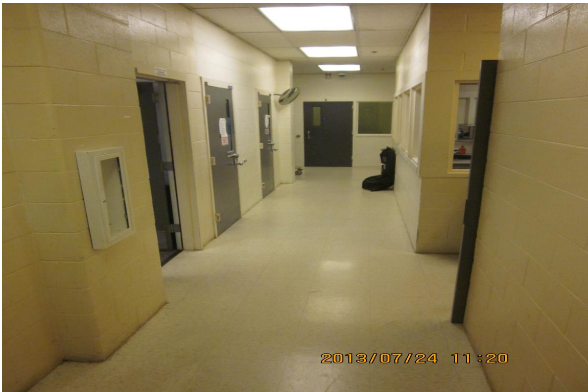
Photo 8. Non-ACM 12-inch beige floor tile and mastic.
