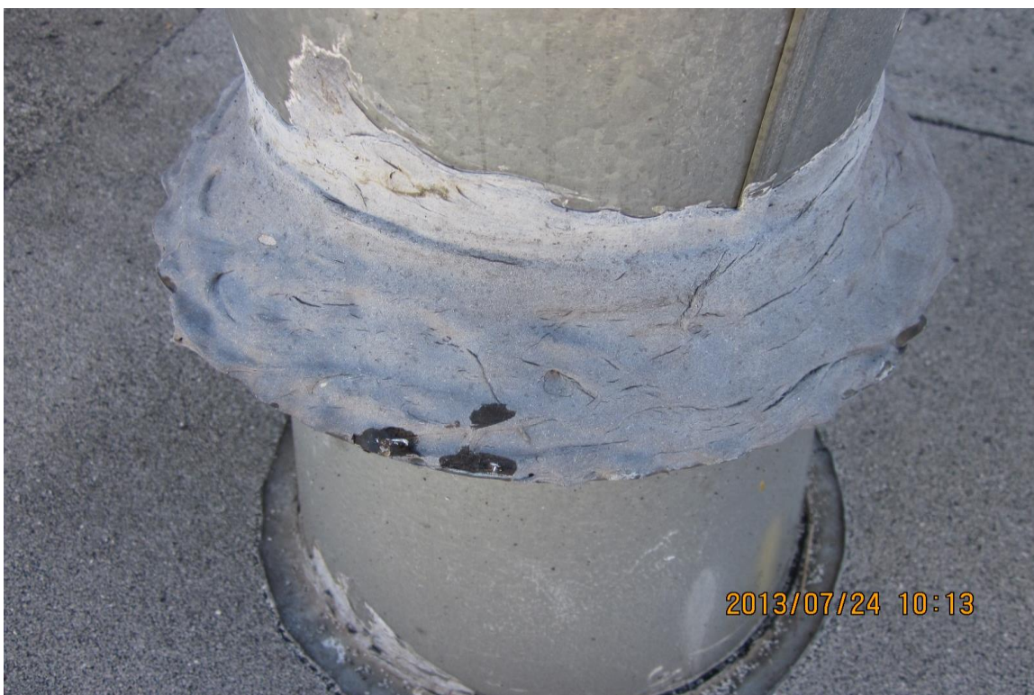
Photo 20. ACM black vent sealant on pool office area roof.
