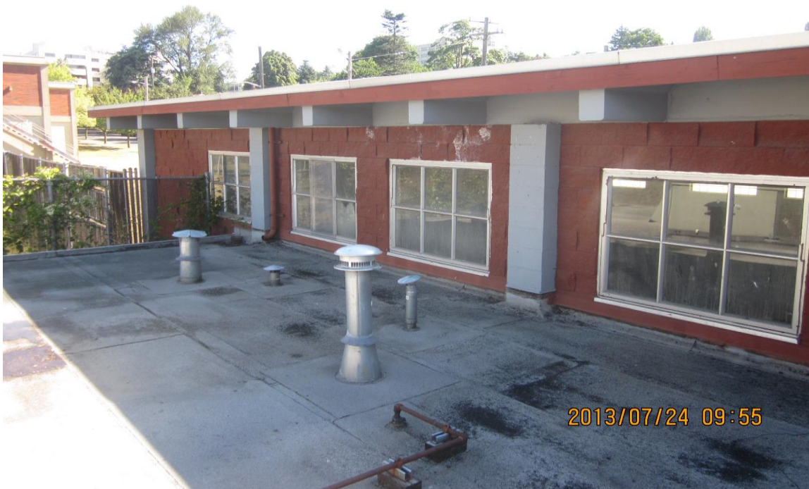
Photo 12. Exterior metal windows on upper pool roof have an ACM black mastic under non-ACM window frame caulk.
