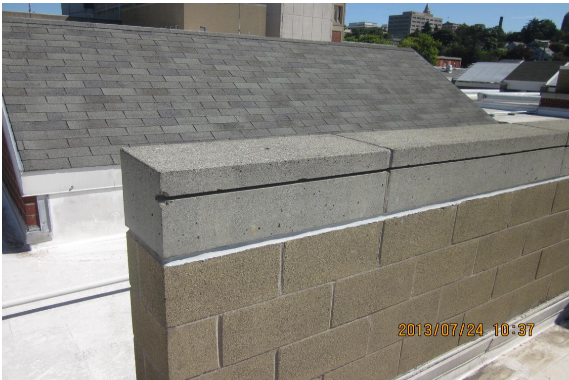
Photo 16. Concrete to CMU wall cap caulk is non ACM. Three-tab composition roofing and vapor barrier is also non ACM.
