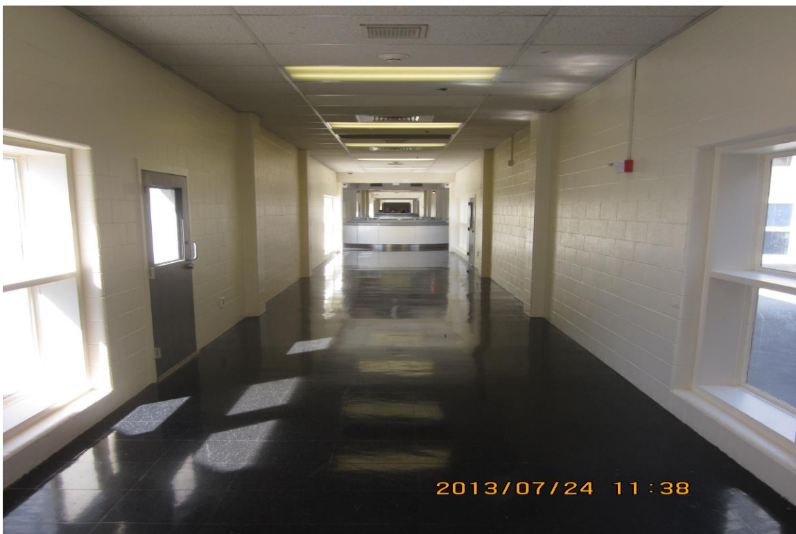
Photo 6. Non-ACM 12-inch black with white flecks vinyl floor tile and mastic.
