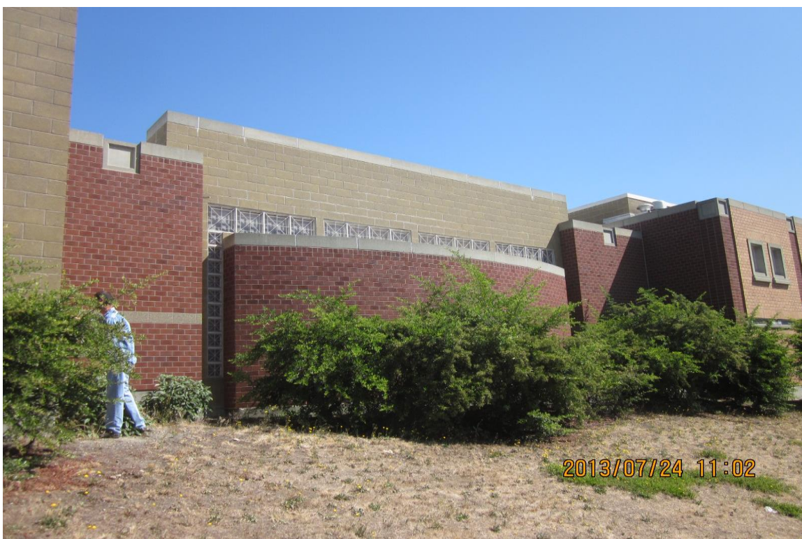
Photo 4. South side of Spruce Wing exterior-concrete and CMU construction with brick finish.
