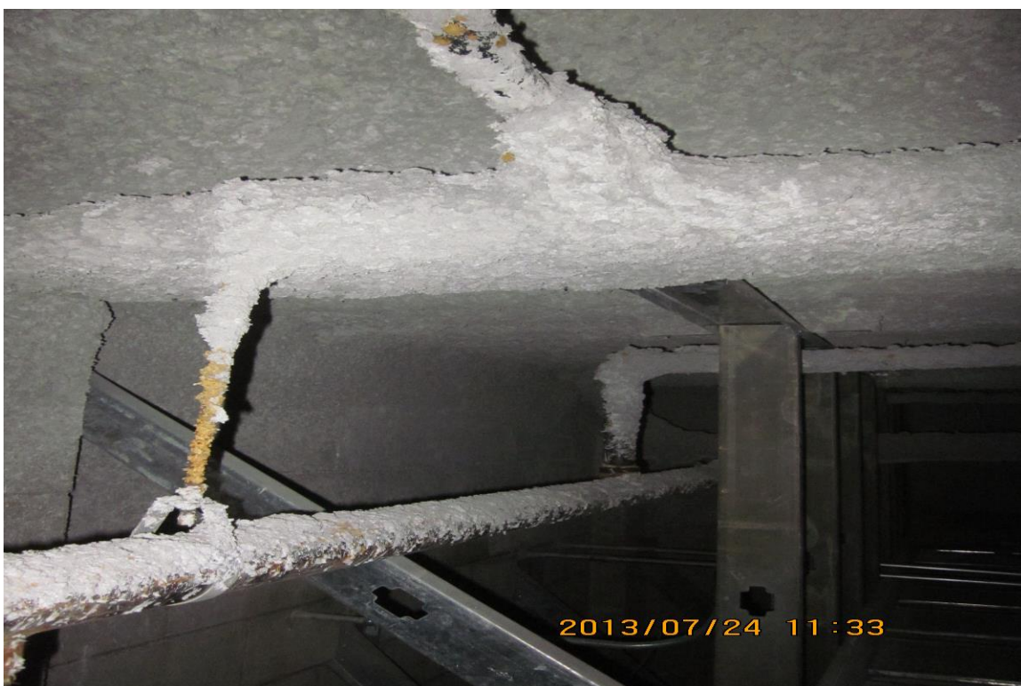
Photo 10. Non-ACM spray-on fireproofing on concrete and steel beams.
