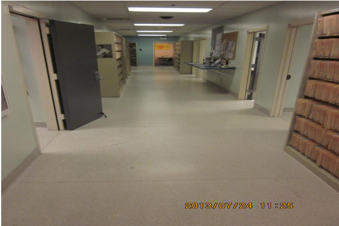
Photo 7. Health Center with Non-ACM terrazzo pattern sheet vinyl flooring.
