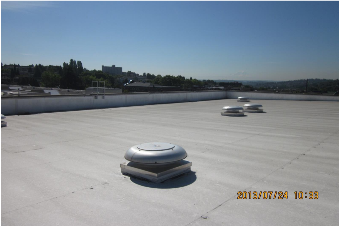
Photo 17. White rubber membrane roofing, tan and gray flashing sealant are non-ACM.
