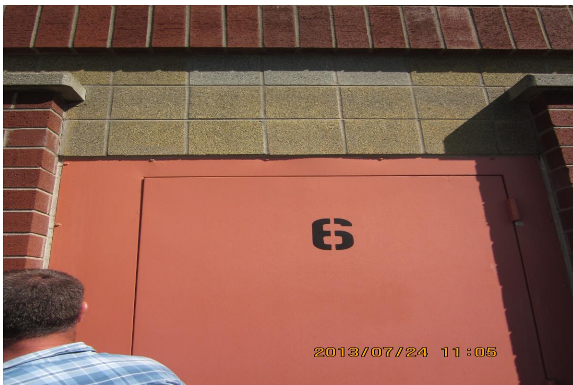
Photo 14. Exterior gray door frame caulk is non-ACM.
