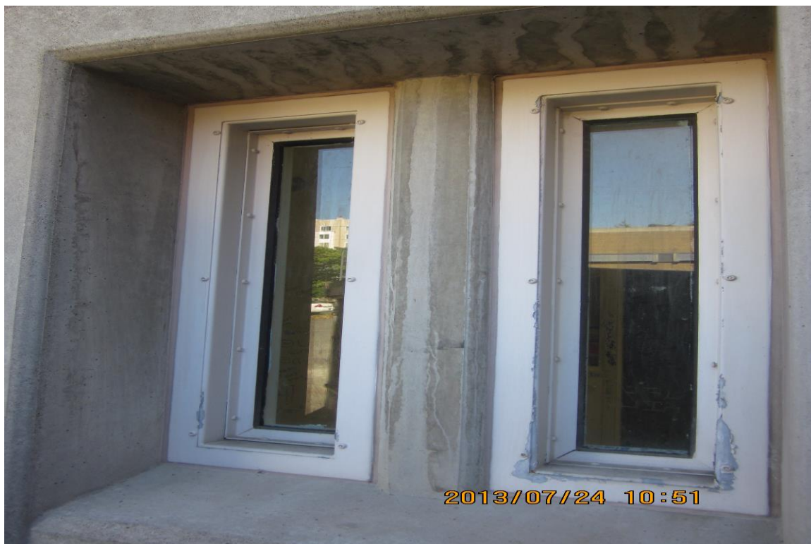
Photo 13. Exterior non-ACM gray window frame caulk.
