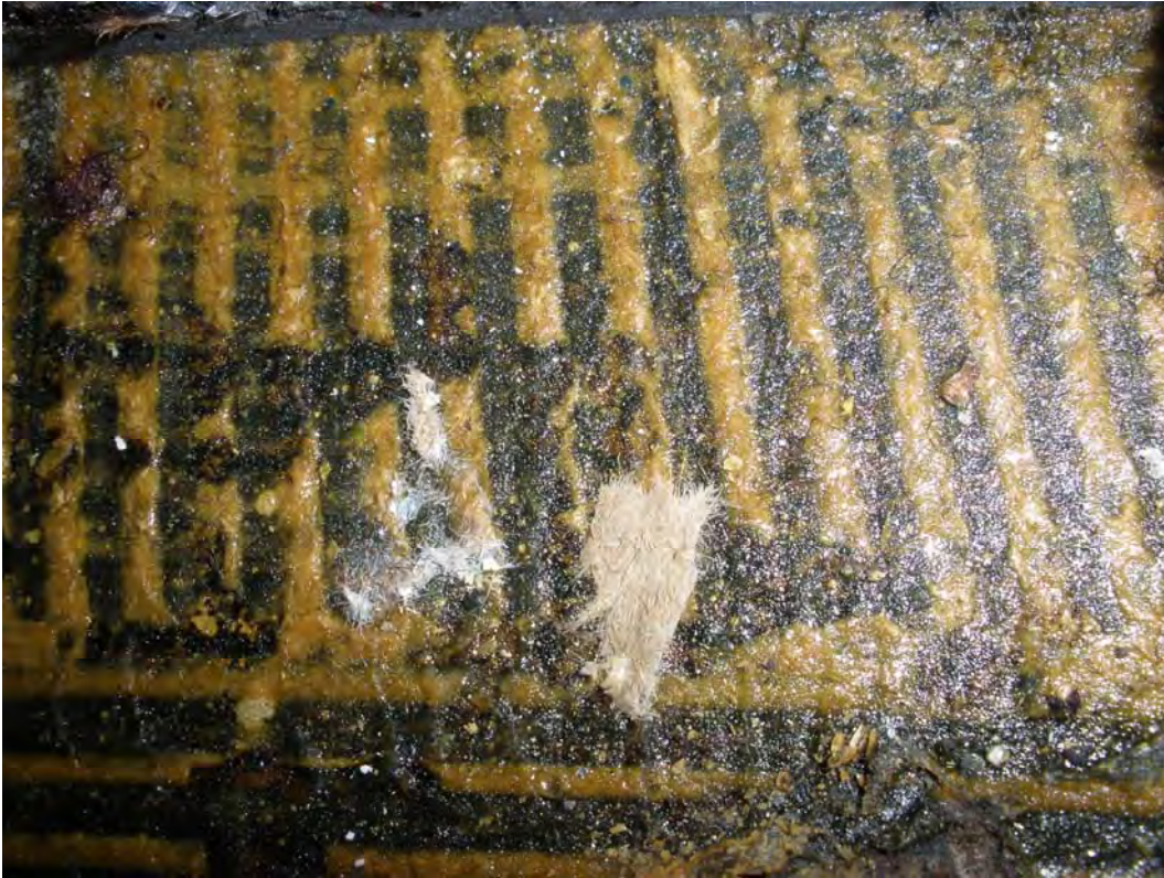
Photo 25. ACM black residual mastic under yellow carpet mastic- 1 st floor Alder Tower
