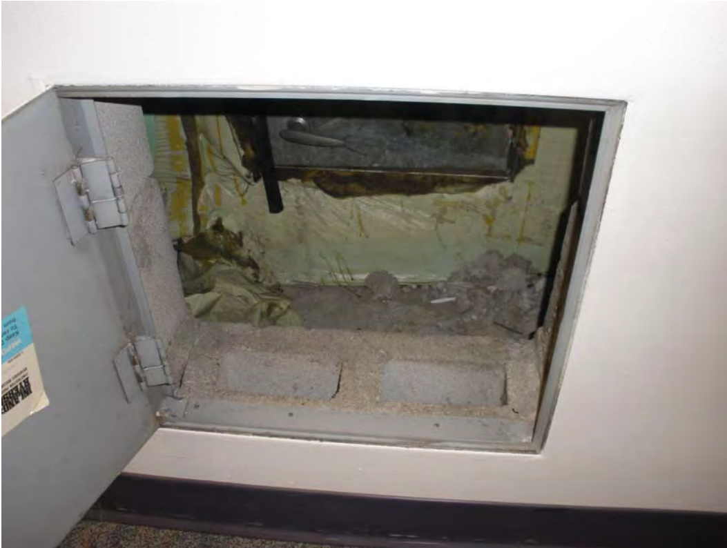
Photo 27. ACM insulating cement on exposed fiberglass pipe insulation ends, roof drain pipe on 5 th floor Alder Tower-interior wall between restrooms
