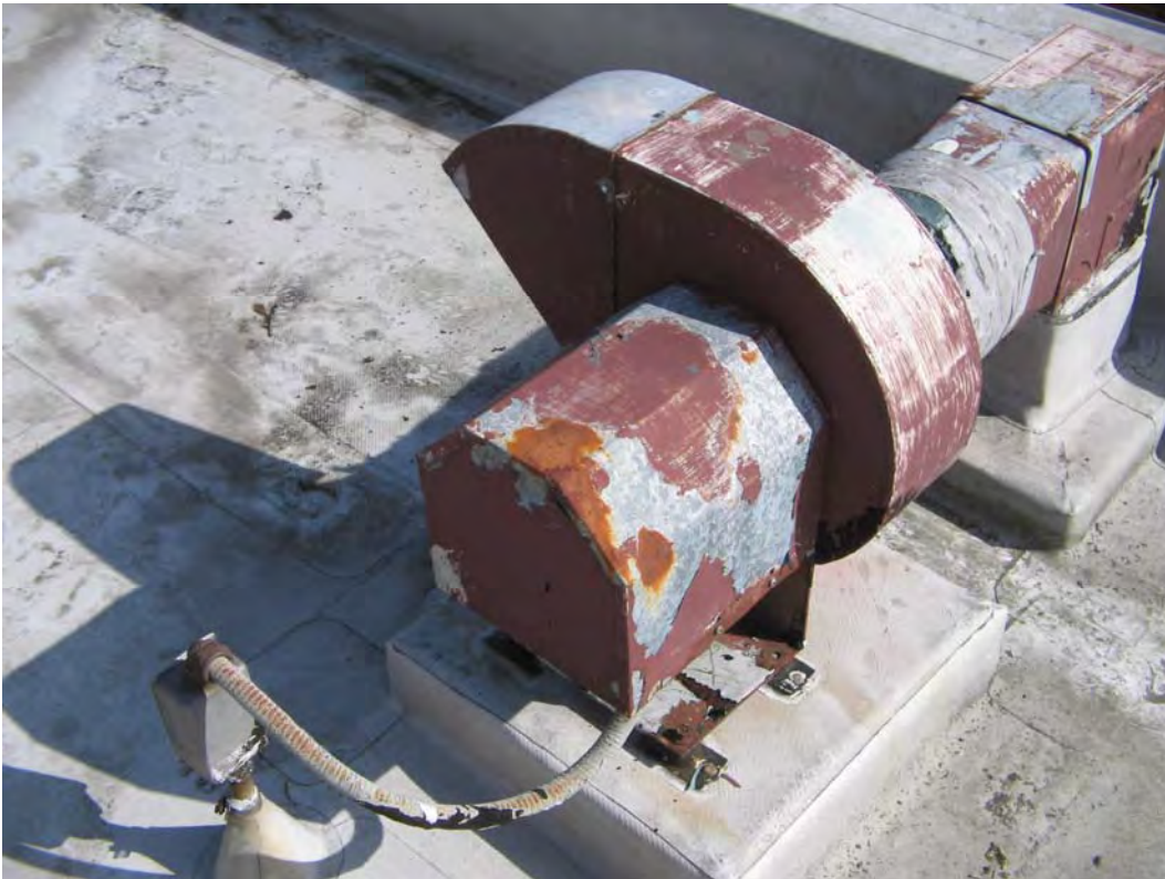
Photo 17. ACM silver paint on reddish brown vent on roof-Alder Tower
