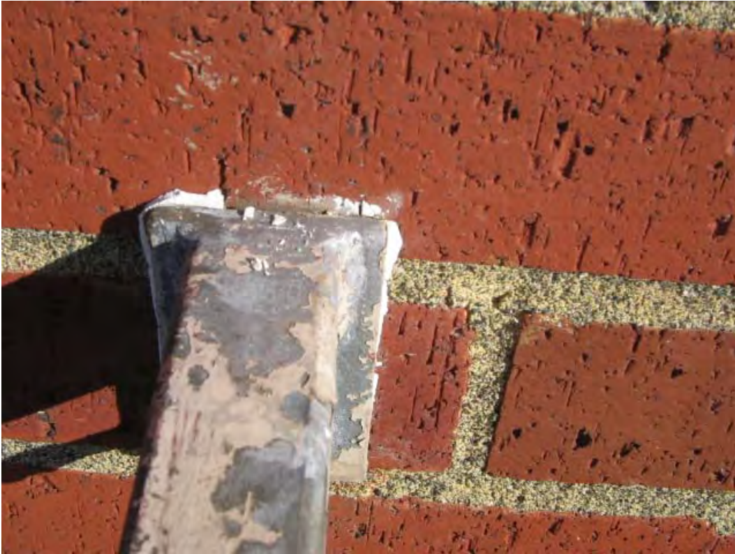
Photo 15. Brick mortar and ACM white rail-to-brick caulking-East Alder wing
