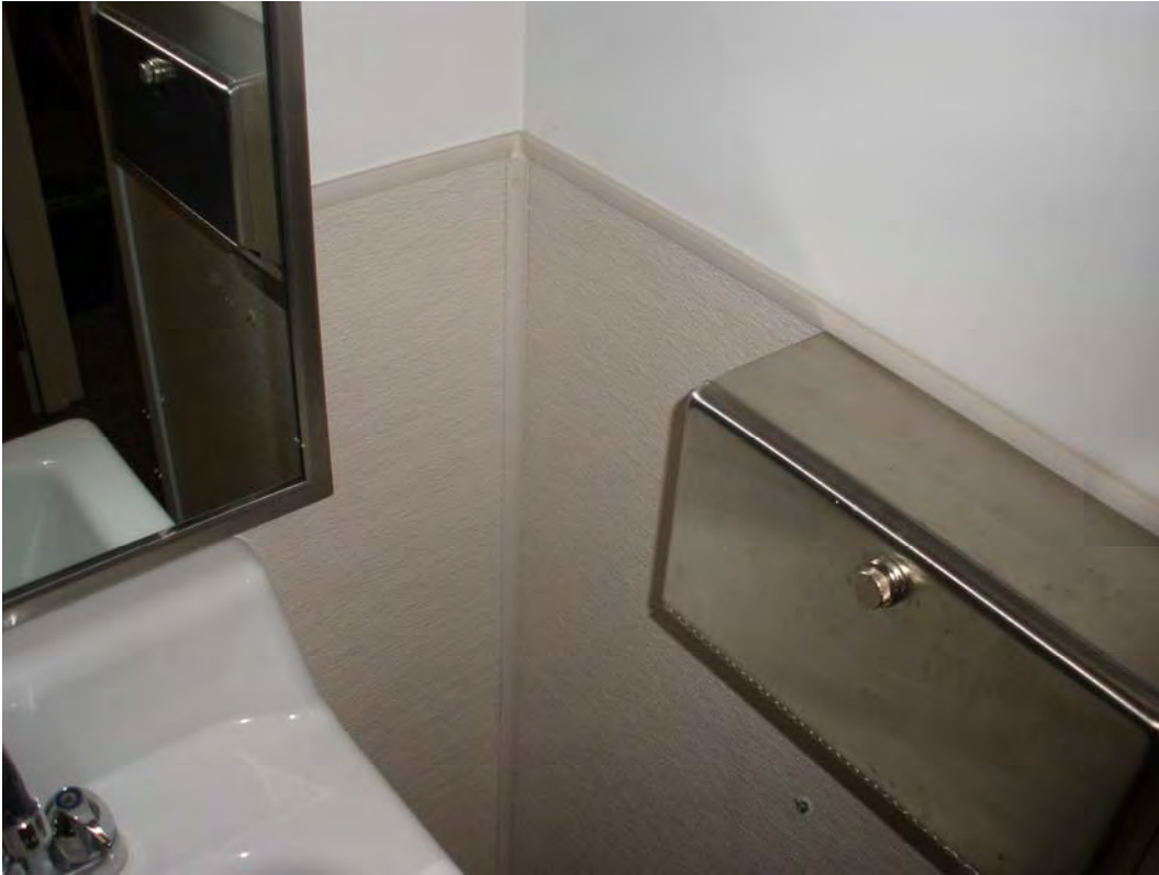
Photo 29. ACM wall panel mastic-Alder Tower main floor Court 3 restroom
