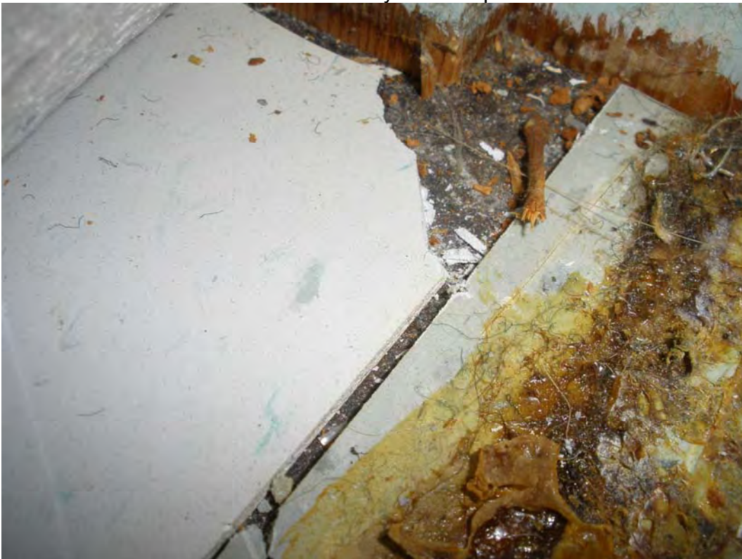
Photo 26. ACM black residual mastic under three types of 12-inch vinyl floor tiles- Alder Tower
