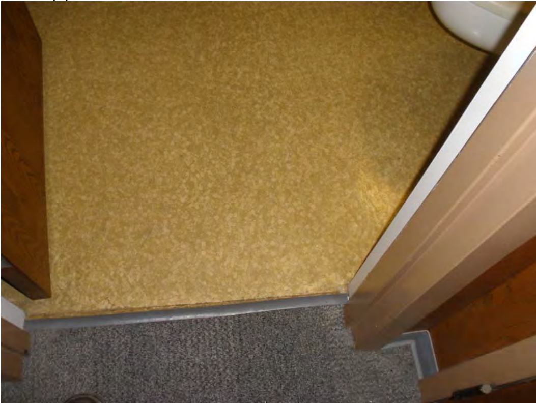
Photo 28. ACM yellow pebble pattern SVF-Alder Tower main floor Court 2-3 restrooms
