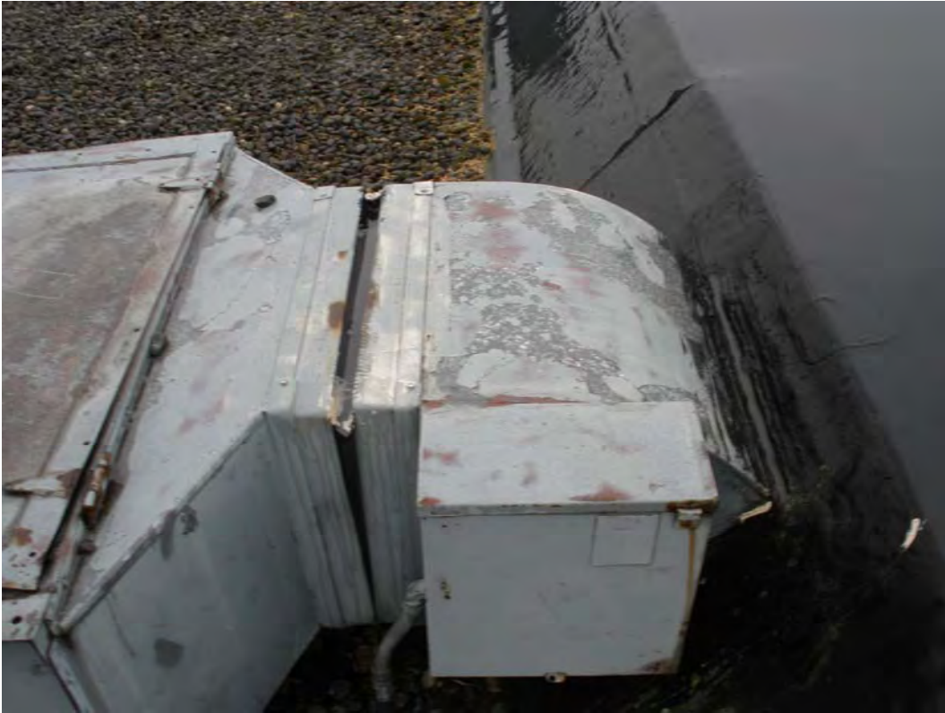
Photo 19. ACM exhaust duct sealant, vent seam sealant, and vent caulk, Alder Wing roof
