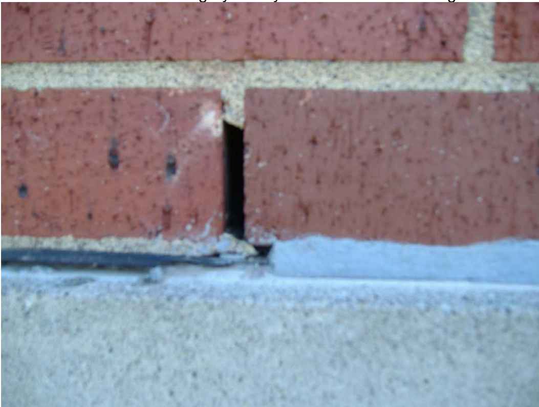
Photo 14. Gray grout with ACM vapor barrier paper (brick to concrete)
