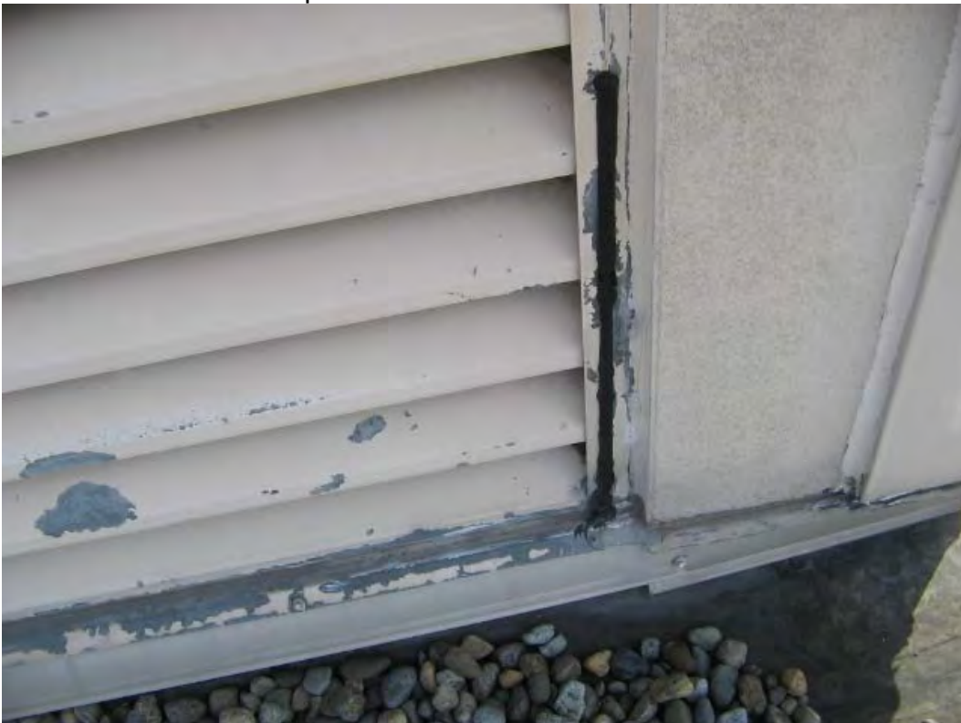
Photo 22. North penthouse of Alder Tower, south wall vent sealants (thin beige and ACM brittle sealant)
