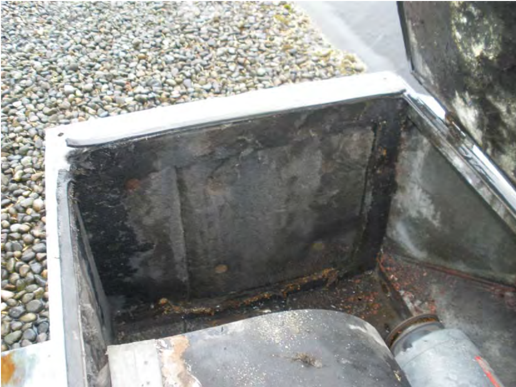
Photo 20. ACM white sealant on vent hatch
