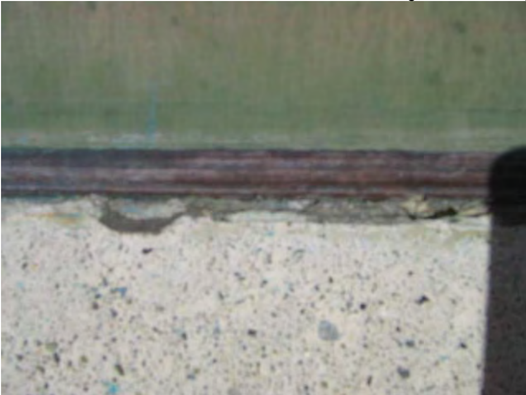
Photo 16. ACM gray window glazing (between concrete and metal) on various exterior Alder wing windows
