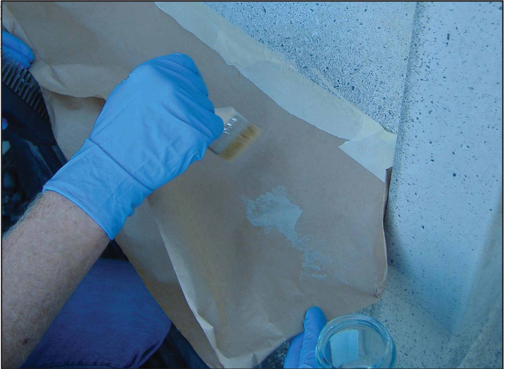
Figure 10. Sealant adjacent to worn area.
