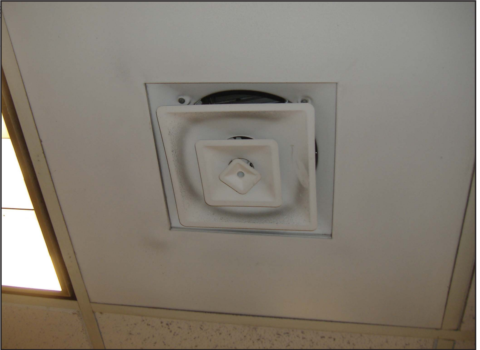
Figure 6. Ventilation cover.
