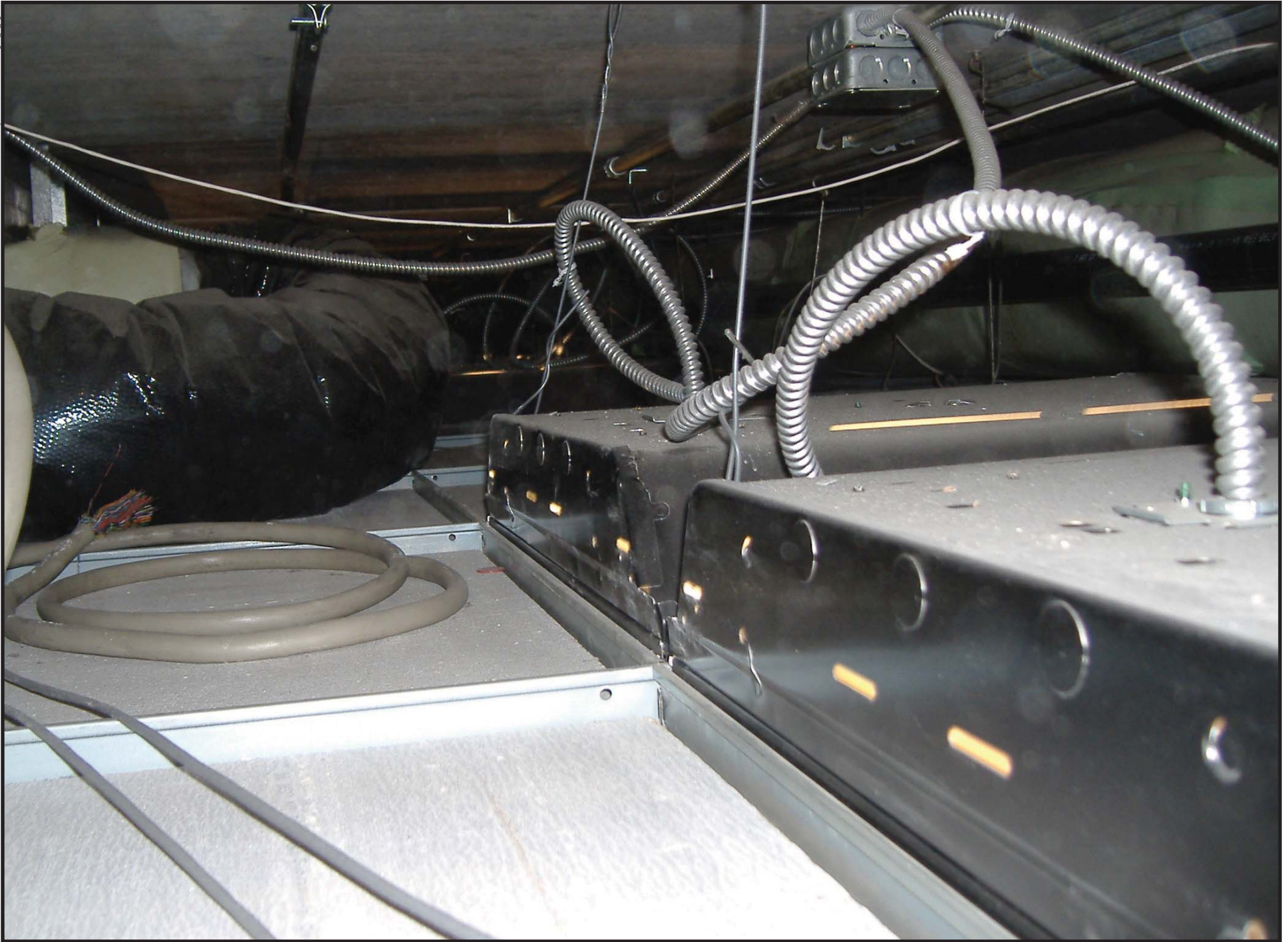
Figure 7. Dropped ceiling space.
