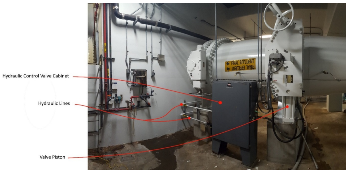
Figure 06. Hydraulic Discharge Valve Assembly
