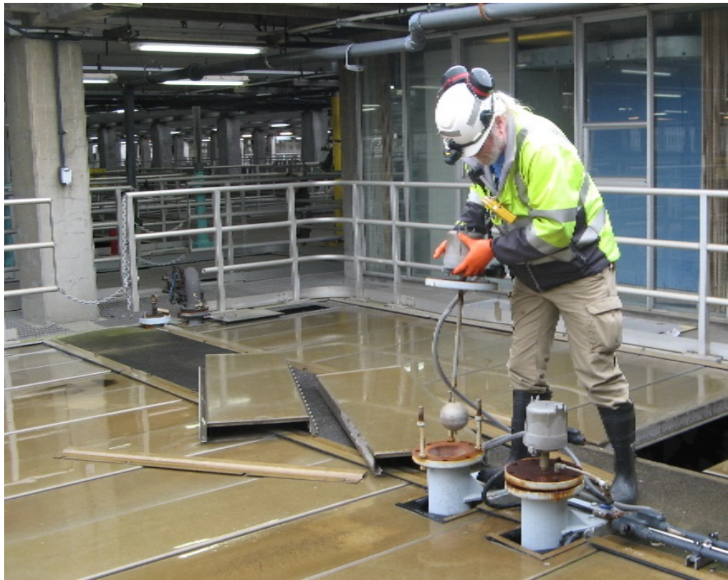
Figure 09. Float Switch Inspection
