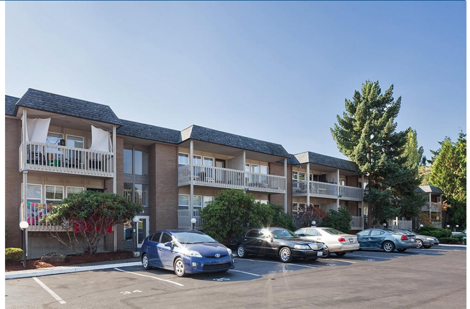
Corinthian Apartments, SeaTac
