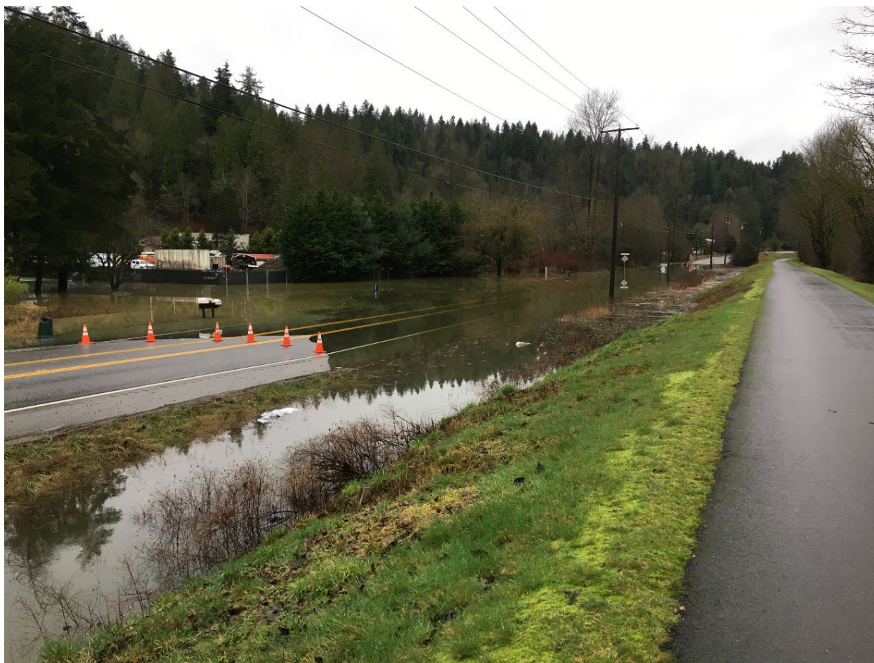
Tributary under State Route 169 flooding from overwhelmed culvert, 2020
