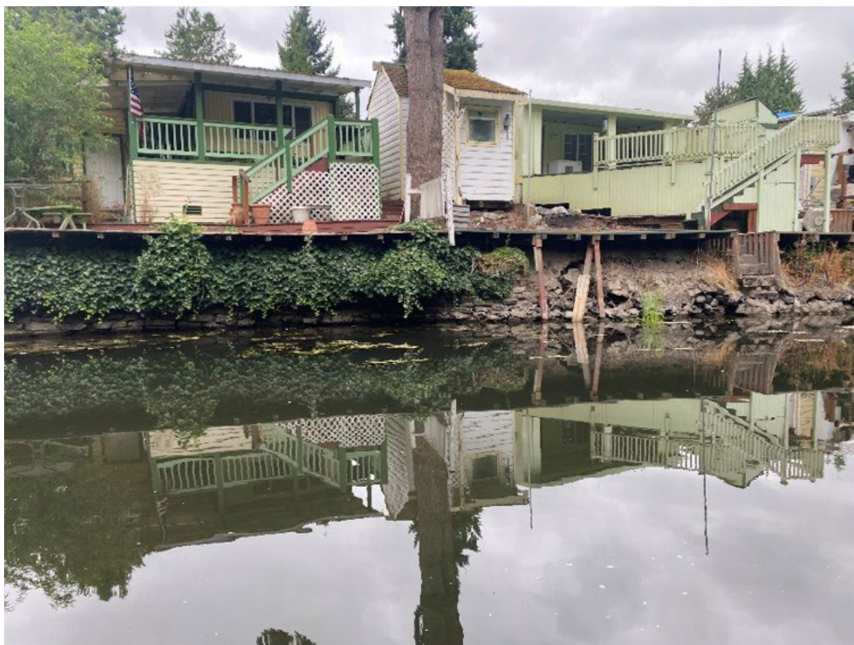
Manufactured home community along the modified banks of the Sammamish River, October 2022
