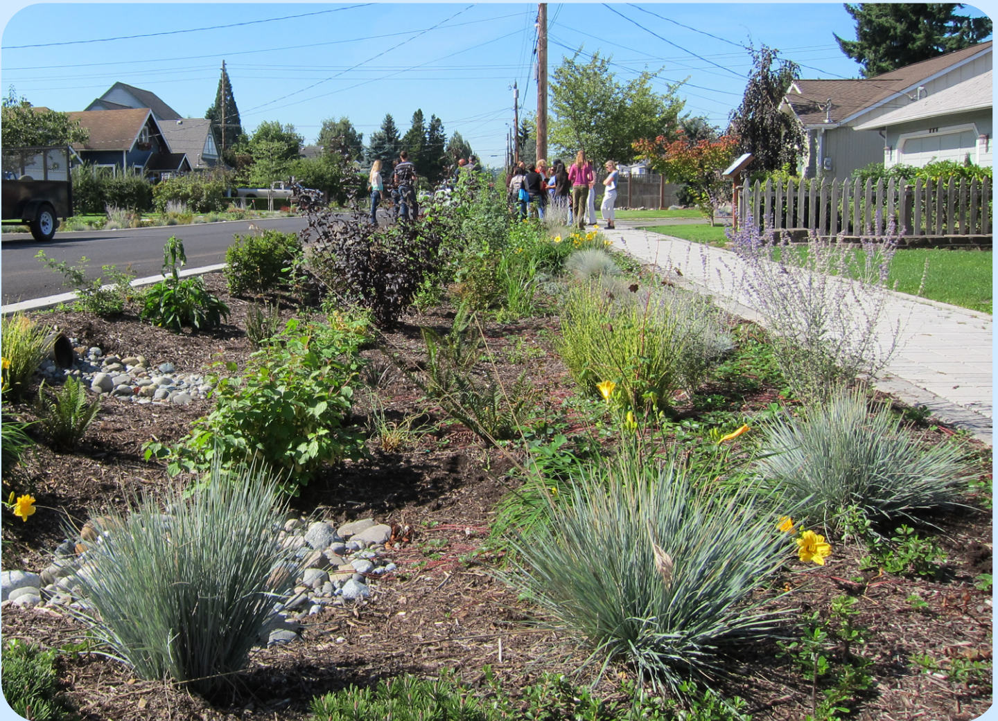
Roadside rain garden for capturing and treating stormwater from streets and sidewalks.
