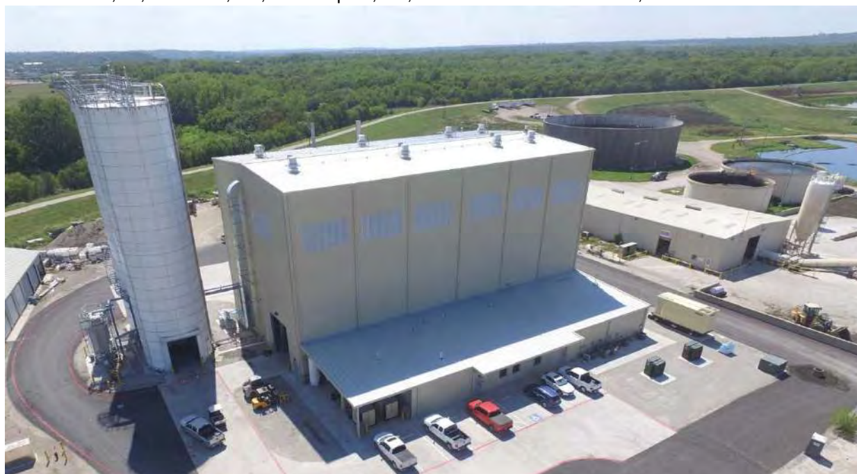
ANDRITZ Biosolids Dewatering and Drying Complex, completed as a Design Build at a cost of $60 million.
