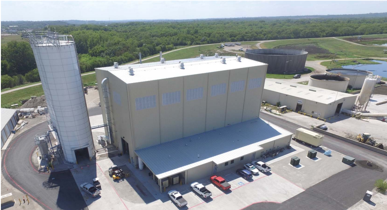
ANDRITZ Centrifuge Dewatering and Drying System 100 dry / 450 wet TPD Commissioned late 2022
