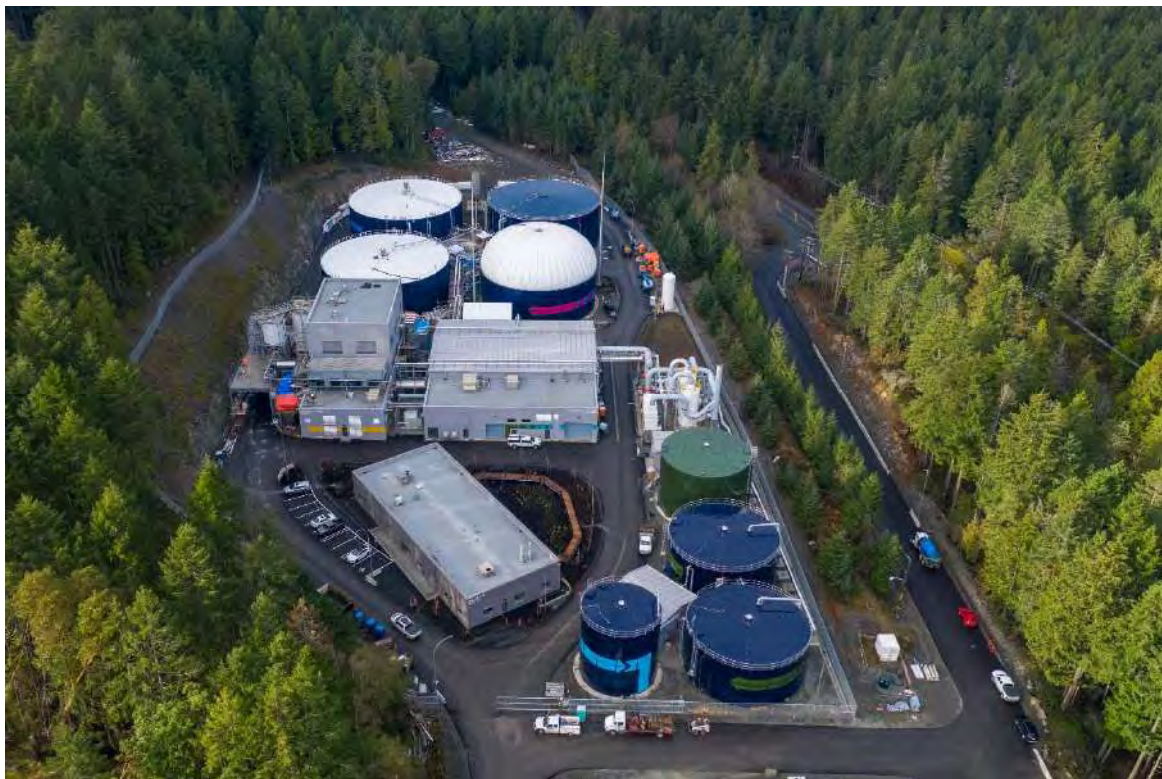
Thickening, Dewatering and Drying buildings centrally located on the site. Odor control to the left
