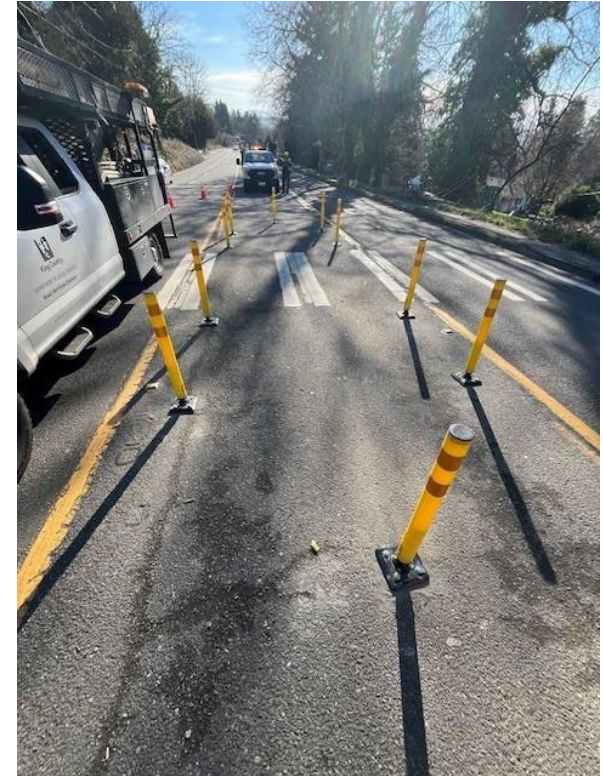
Roads installed 13 traffic calming “islands” on Renton Ave to calm traffic and prevent unsafe passing
