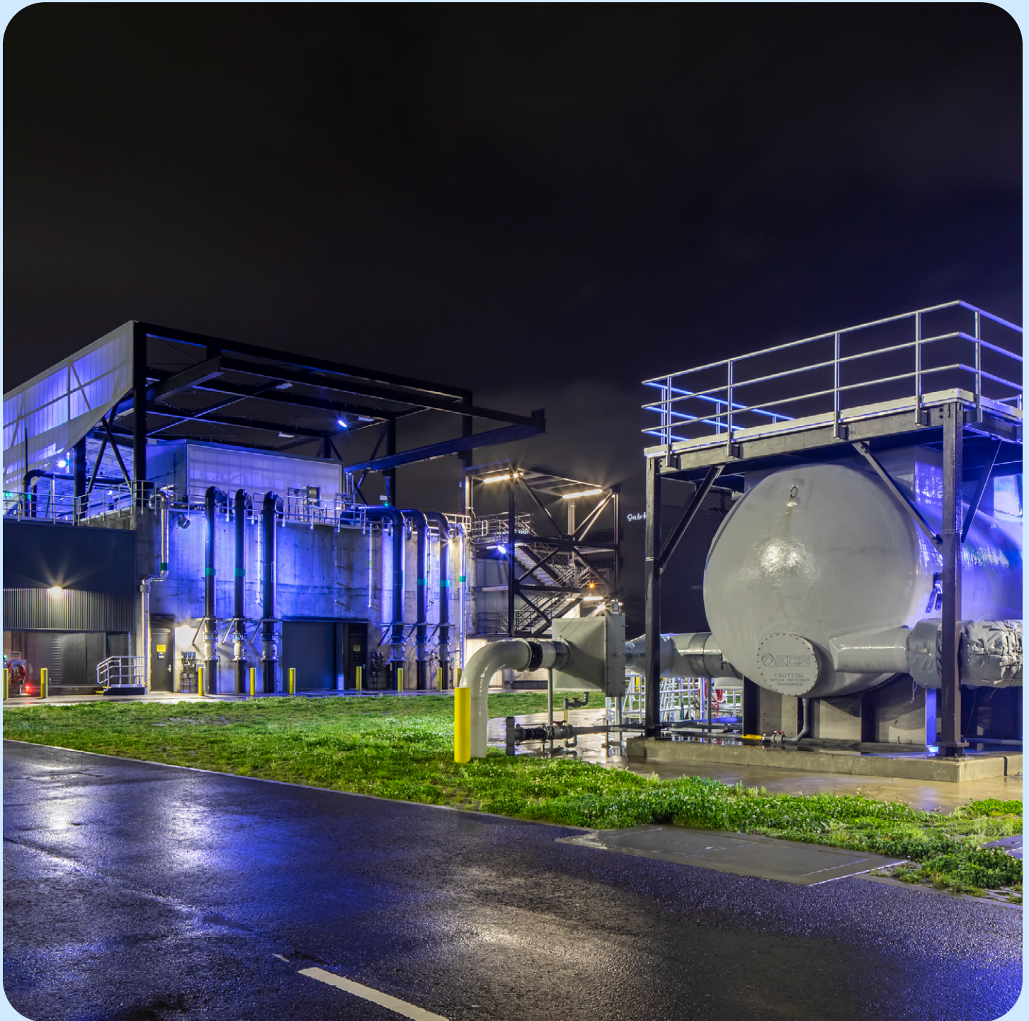
King County's Georgetown Wet Weather Treatment Station, located in Seattle's Georgetown neighborhood. The station was designed to account for two feet of sea level rise.
