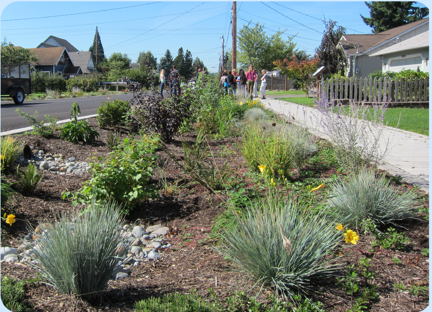
Roadside rain garden for capturing and treating stormwater from streets and sidewalks.
