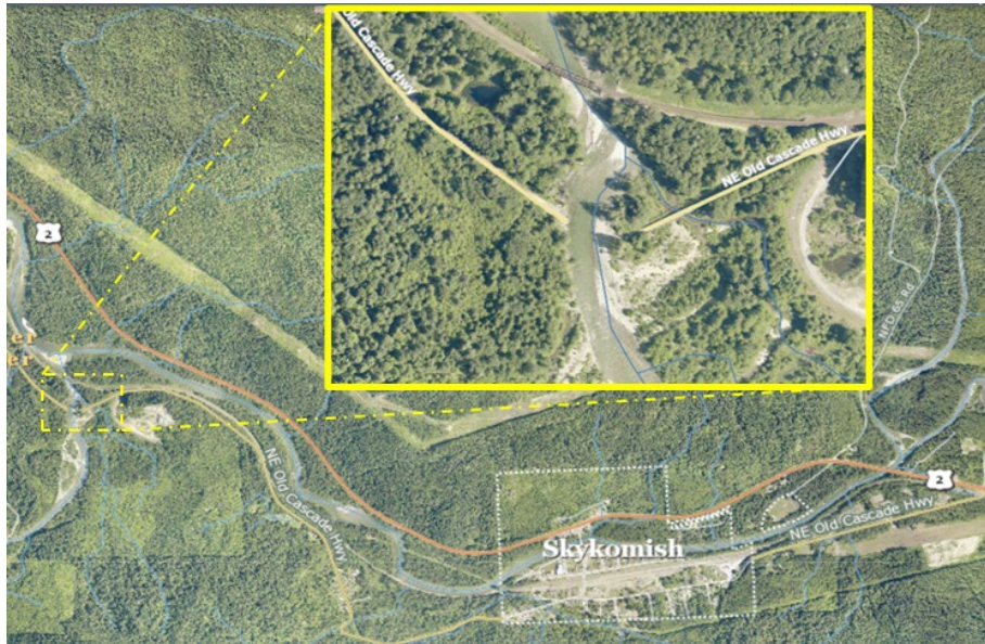
Figure 3 – 2021 Aerial View with Inset of Miller River Bridge and Washed-Out Approach
