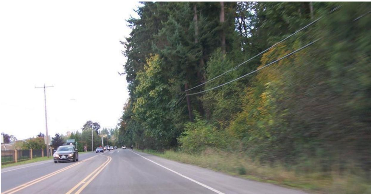
The following photo shows a low make-ready pole line that has only one existing attachment in the communications space. Where make-ready is low, the cost of aerial construction is cheaper than in high make-ready areas.
