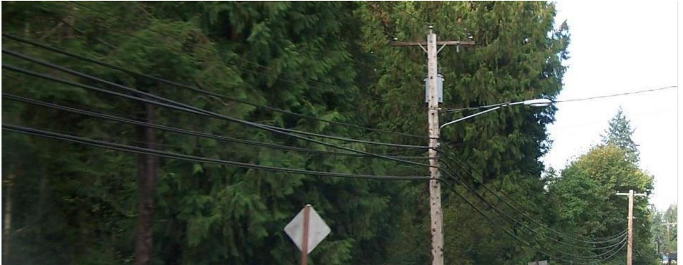
Tree trimming is required to attach an additional attachment on the utility poles in the following picture. Tree trimming is also an important maintenance function necessary to keep the pole line clear of tree limbs that could break and damage the wires on a utility pole.
