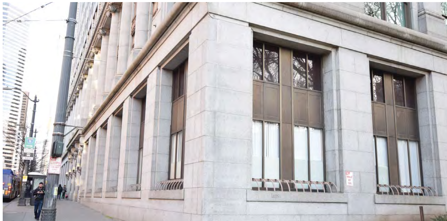
King County Courthouse exterior, view of the aluminum window wall systems at the southwest corner of the first floor. CDG photo, March 18, 2016.
