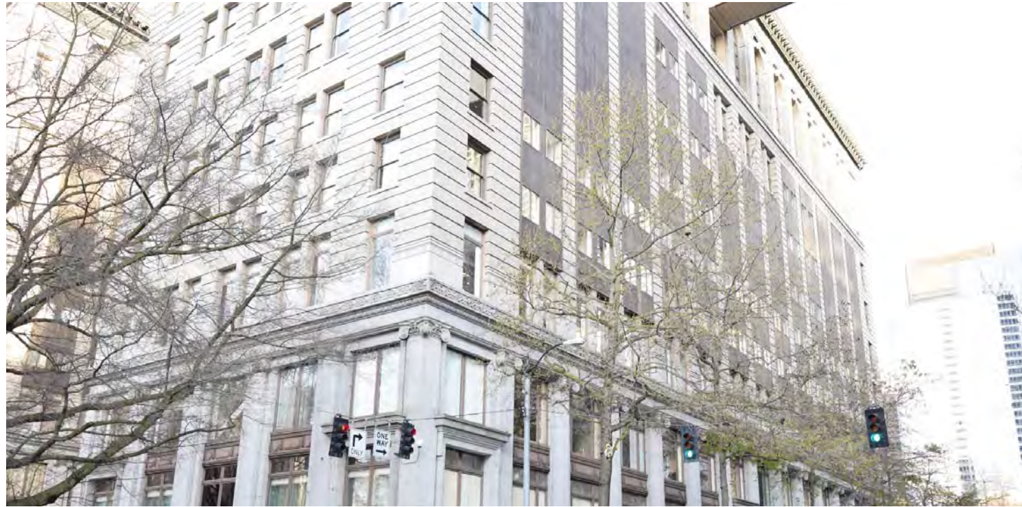
King County Courthouse exterior, view of the aluminum window wall systems at the Fourth Avenue facade. CDG photo, March 18, 2016.
