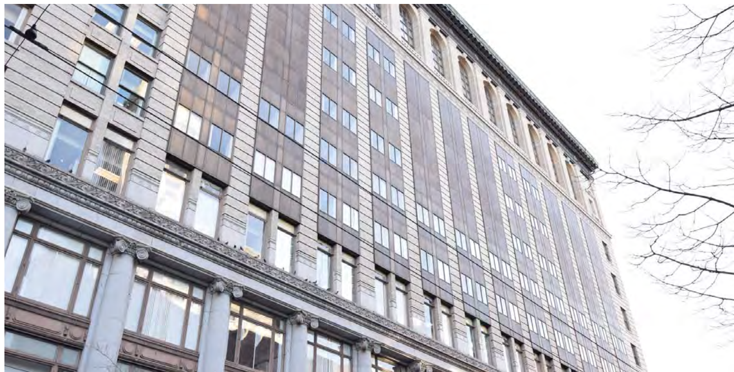
King County Courthouse exterior, view of the aluminum window wall systems at the Third Avenue facade. CDG photo, March 18, 2016.
