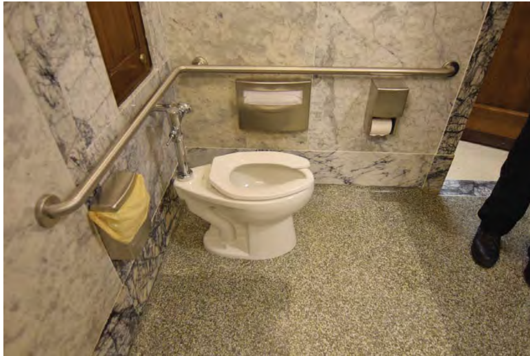
King County Courthouse jury deliberation room restroom E761B showing the ADA upgrade performed by King County Facilities Management Division. CDG photo, June 2, 2016.
