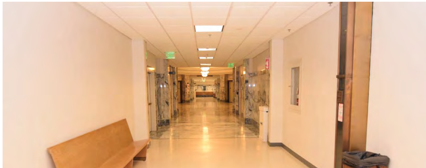
Fluorescent lighting in typical corridor
