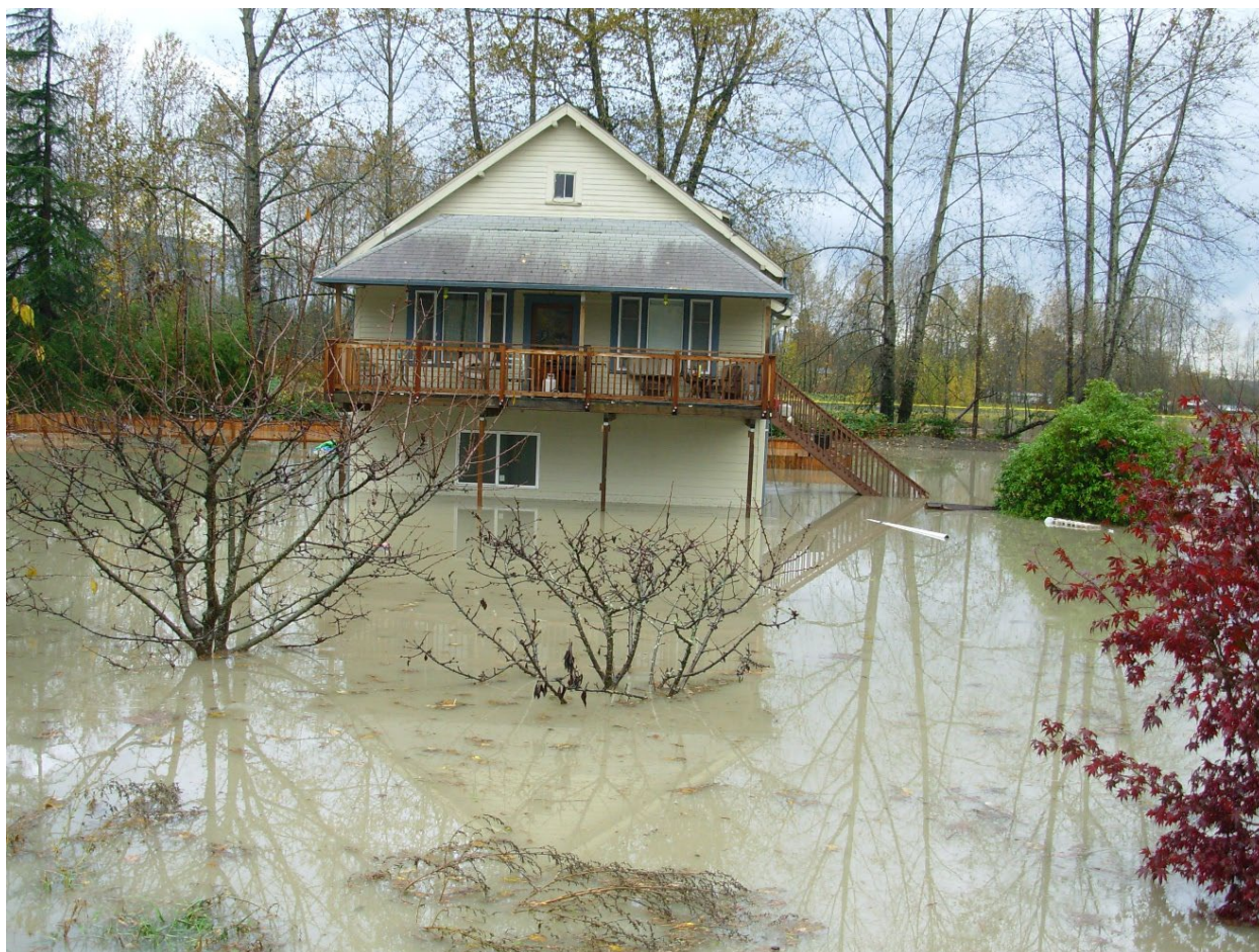
Elevated home in Snoqualmie River Watershed during floods, November 2006
