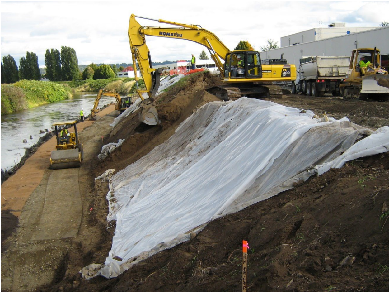
Briscoe Levee construction on the Green River, September 2007
