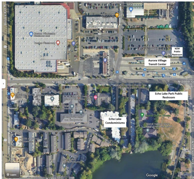
Figure 3 Aerial View of Aurora Village Transit Center Figure 4 Aerial View of Burien Transit Center
