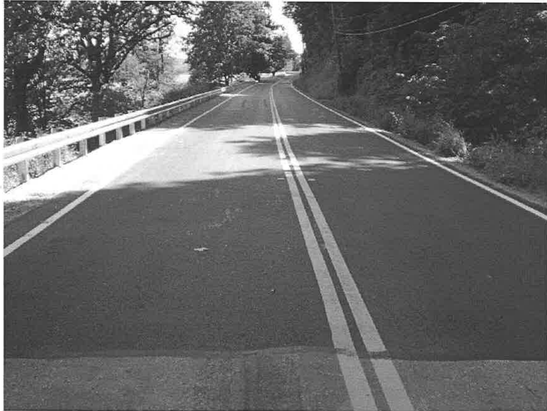
West Snoqualmie Valley Road
