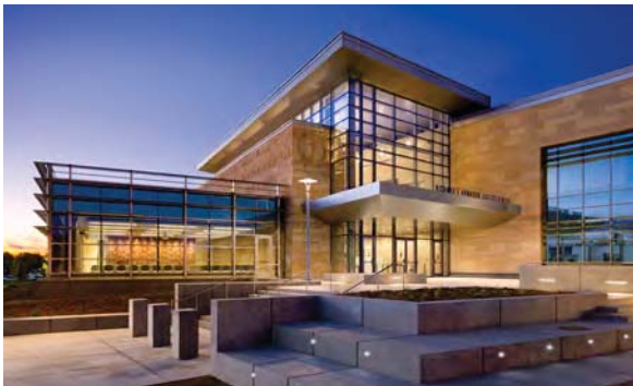
The jury assembly, traffic court, and entry lobby portion are carefully planned to be isolated from the rest of the facility for after-hours use for night court or the community.
