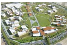
San Diego Women’s Detention Facility
