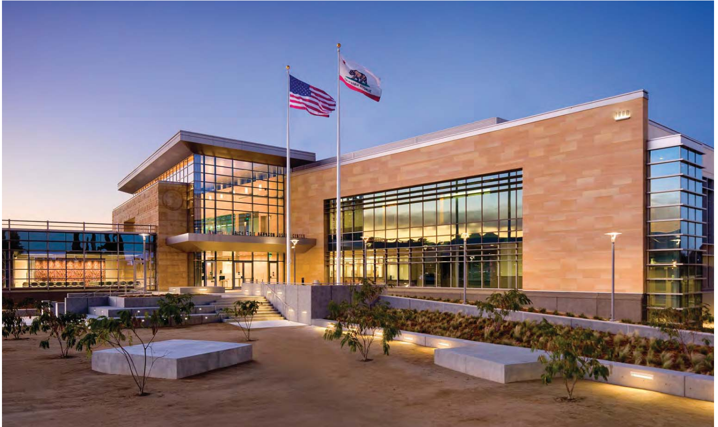
The court's monumental limestone facade presents a sense of dignity, while welcoming visitors with transparent public spaces.
