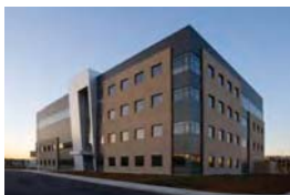
US Coast Guard Shore Ops & Admin Building
