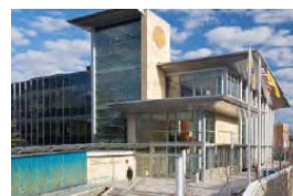
Gloucester County Justice Complex
