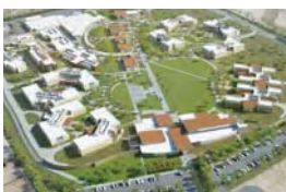
San Diego Women’s Detention Facility
