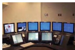
King County Corrections Facility
