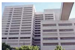
King County Corrections Facility
