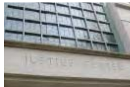
Multnomah County Detention Facility
