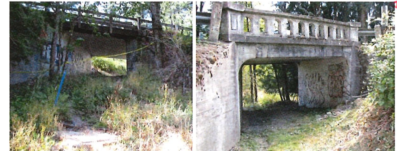
EXISTING BRIDGE/TUNNEL IN PRESTON-FALL CITY ROAD
