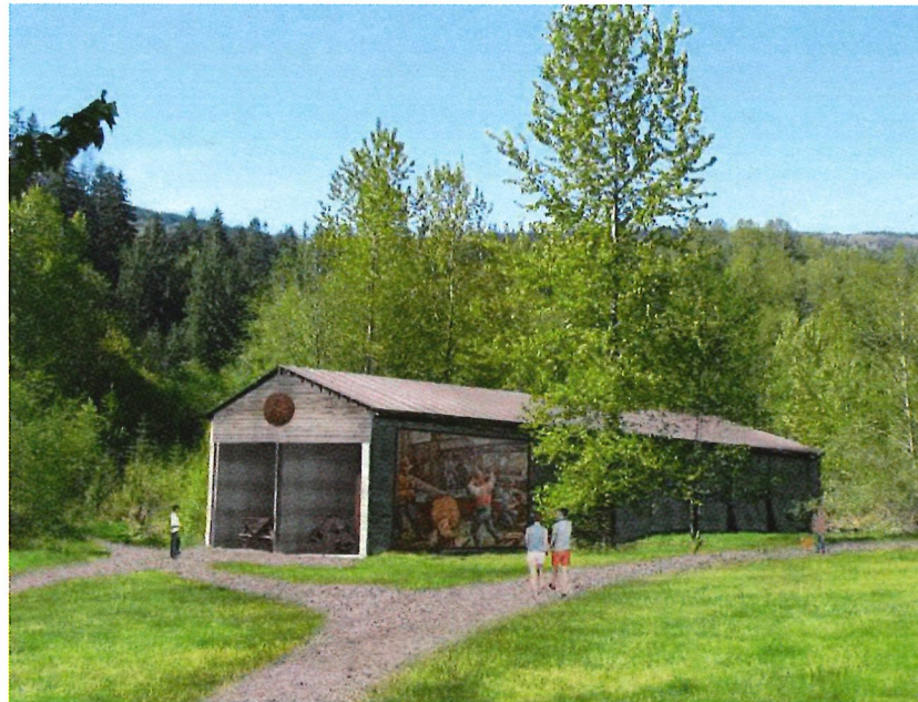
SIMULATION OF REPAIRED KILN BUILDING TO BE MAINTAINED AS HISTORIC RELIC WITHOUT INTERIOR ACCESS AND USE
