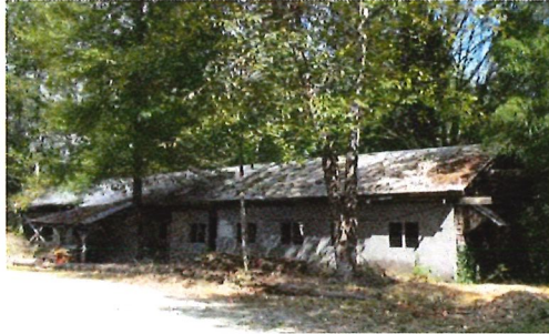
EXISTING MILL SHED BUILDING (TO BE REMOVED)
