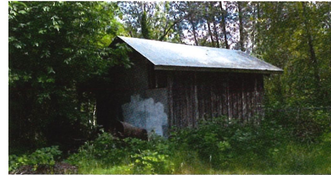
EXISTING SMALL SHED BUILDING
