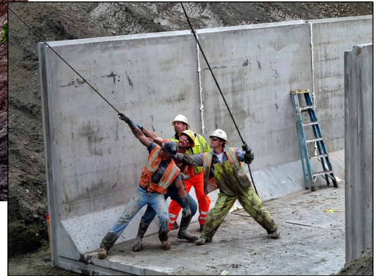
June 2011: Workers strain under the weight of a huge concrete culvert section being placed in a deep trench beneath SR 520.
