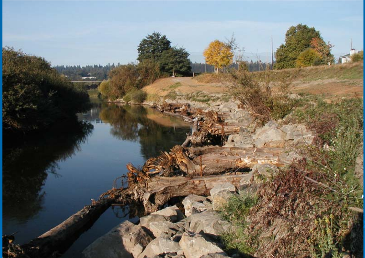
Bio-engineered levee setback - Lower Green River
