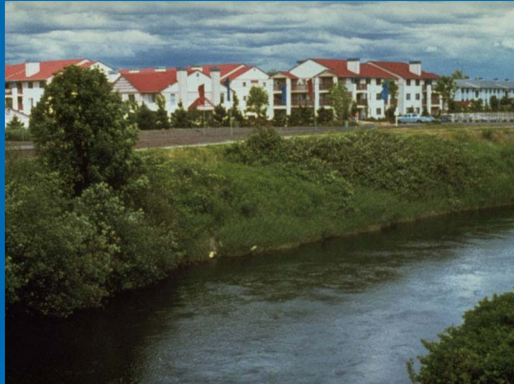
Lower Green River levees
