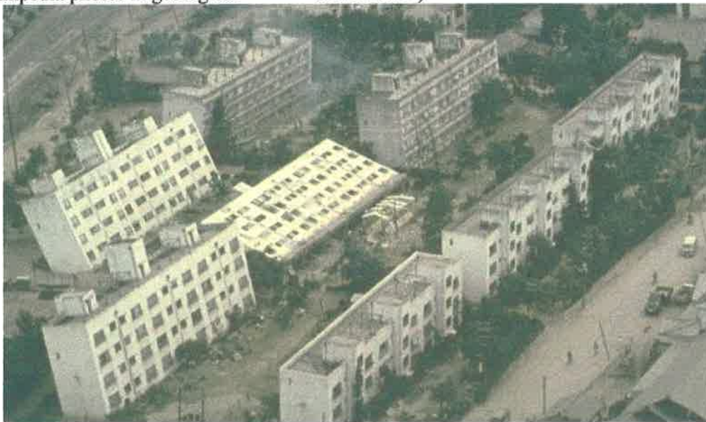
3/26/'19 Map 2: Photo 7: Liquefaction at Niigata Japan 1964 (source: WIKIPEDIA on subject Liquefaction). Liquefaction danger increases with soil fill, water, & disturbances (vibration, earthquakes, etc.).
