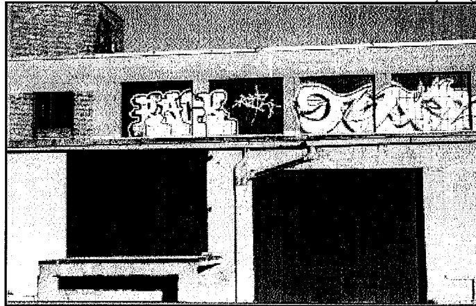
Graffiti often appears in hard-to-reach yet highly visible locations, such as on the upper-story windows of this warehouse.
