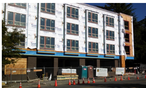
Construction is underway at DESC Delridge. Photo by Kimberly Cisson.
