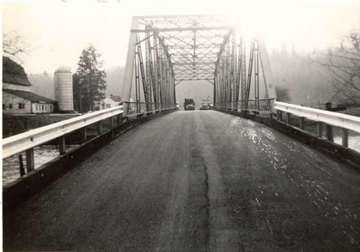
Whitney Bridge, looking south from Green Valley Road, c. 1930 Courtesy of King County Archives.
