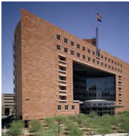
Phoenix Municipal Courthouse
