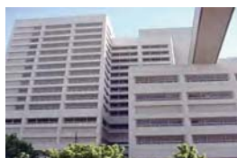
King County Corrections Facility
