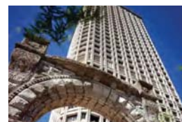
Jackson Federal Building
