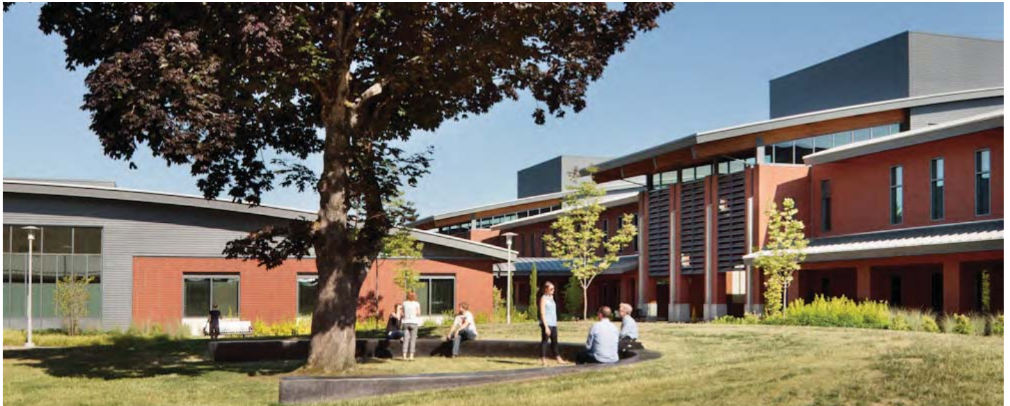
The HOK design team was challenged to create a hierarchy of spaces and prioritize them based on activities that happen in each space, creating a functional pathway based on the needs of residents and staff.
