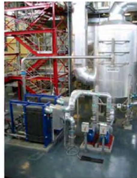
Spray Condenser with heat recovery pumps and heat exchangers (up to 75% heat recovery as hot water)
