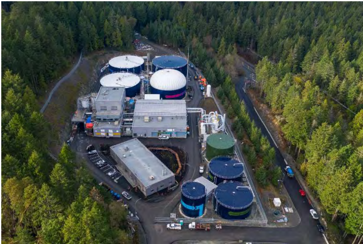
Thickening, Dewatering and Drying buildings centrally located on the site. Odor control to the left
