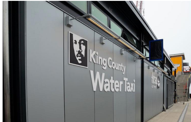
Figure 8- View of the new Pier 50 facility
