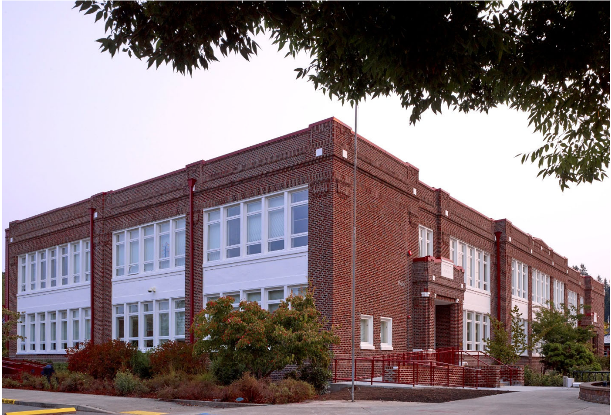
Old Redmond Schoolhouse – Opened Fall 2020
