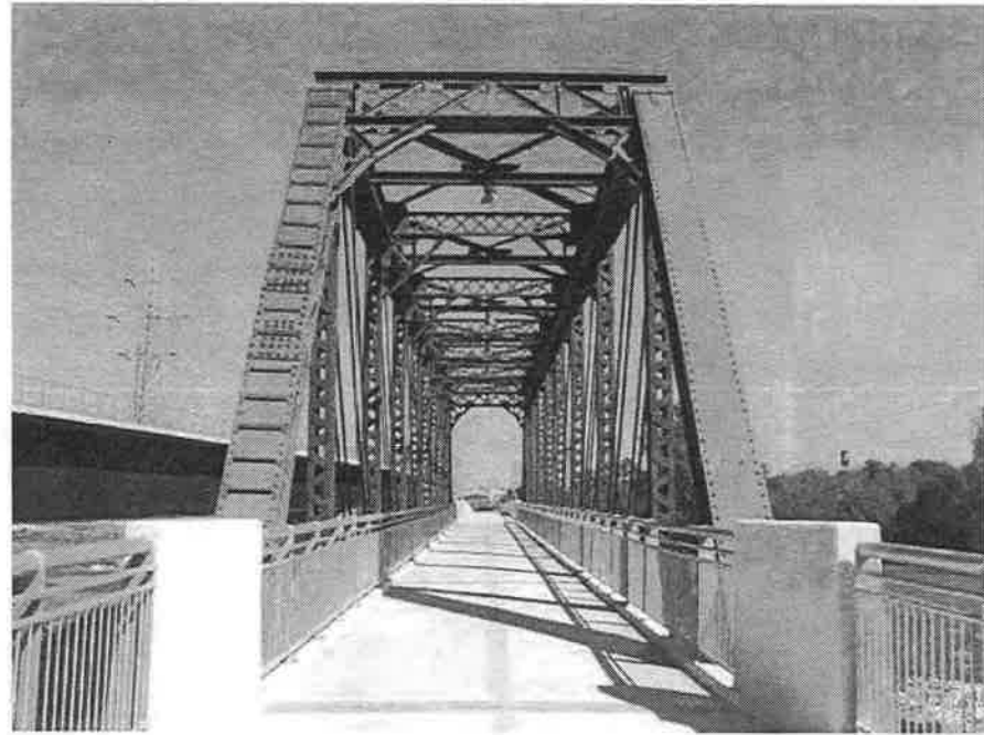
Santa Fe Trestle – Santa Fe, NM
