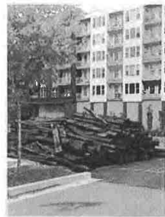
Mixed use residential developments abutting the Downtown section of the ERC.
