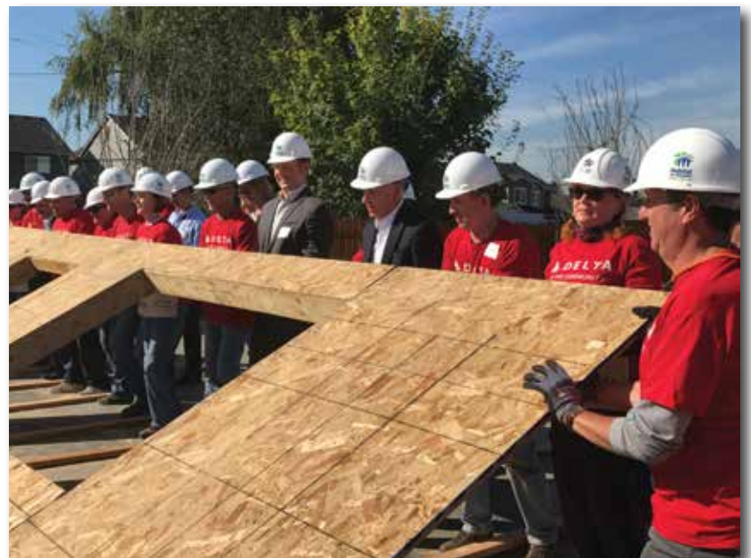
Raising the wall for one of nine Habitat for Humanity Blitz Build homes for veterans in Pacific.
