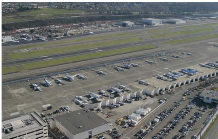
King County International Airport
