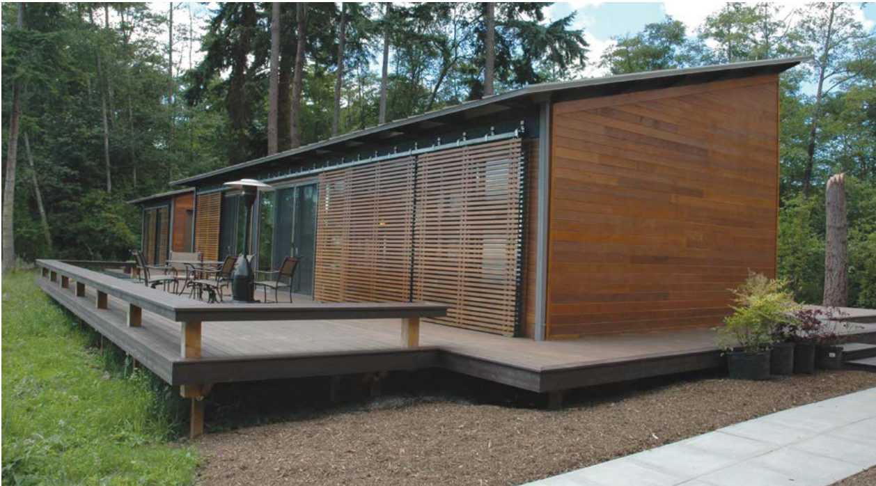
The Glidehouse is a net-zero energy home located on Vashon Island in unincorporated King County.
