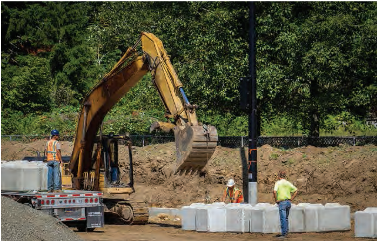
Preston Ballfields Construction
