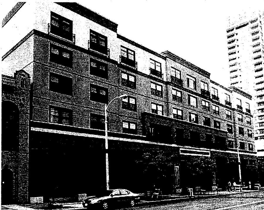
The Langdon and Anne Simons Senior Apartments developed by Plymouth Housing Group and supported by the levy was recently named a finalist in Affordable Housing Finance Magazine's Fifth Annual Reader's Choice Award for the nation's best low-income housing developments in 2008.
