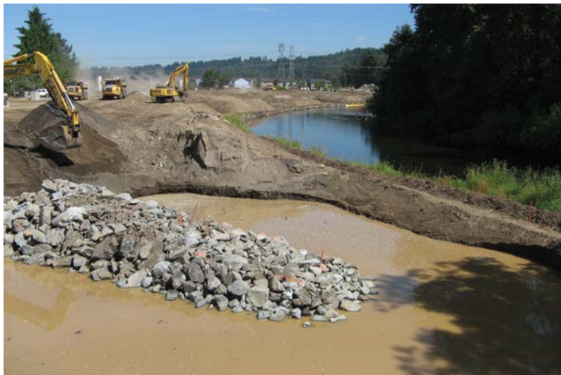
The creation of the Flood Control District has resulted in a substantial increase in local funding for flood risk reduction activities, with 2015 tax revenues of $52.8 million. Pictured here is the Reddington Levee setback project along the Green River in the City of Auburn.
