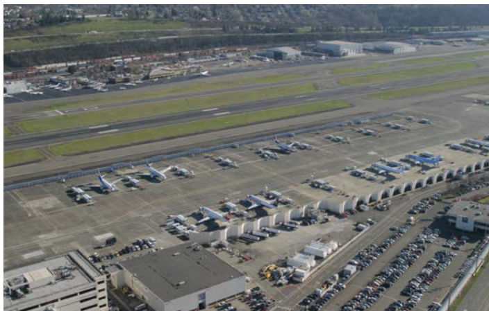
King County International Airport
