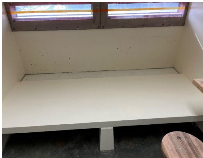
Figure 7: Retrofitted bunk at KCCF, showing infill between the bunk surface and wall
