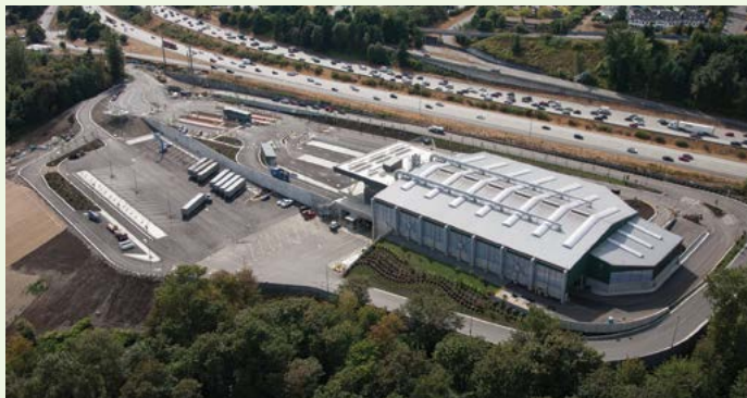
Solid Waste Division’s Bow Lake Recycling and Transfer Station located in Tukwila achieved a LEED Platinum level certification featuring renewable energy, water reclamation and reuse system, and Forest Stewardship Council (FSC) certified wood.
