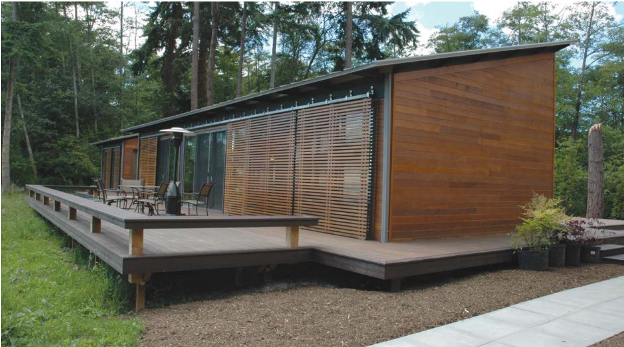
The Glidehouse is a net-zero energy home located on Vashon Island in unincorporated King County.
