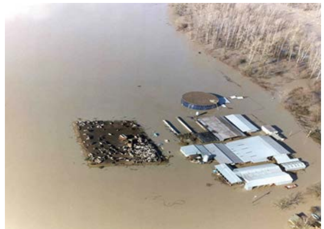
As the service provider for the King County Flood Control District, King County supports the construction of farm pads like this one, near a flooded Snoqualmie River in 2009, which protects farm equipment and animals.
