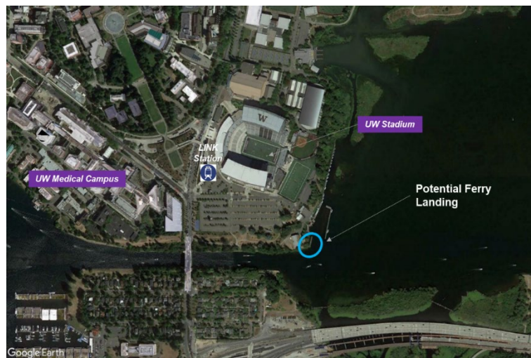
Figure 6: Aerial View of the UW WAC and Surrounding Area (Google Earth)
