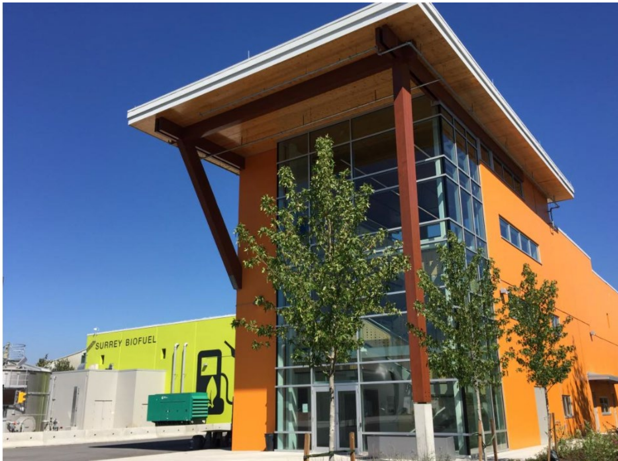
Figure 3-17. City of Surrey biofuel facility
