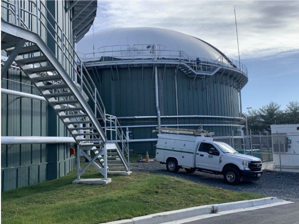
Figure 3-6. Bioenergy Devco low-solids AD tank, Jessup, Maryland
