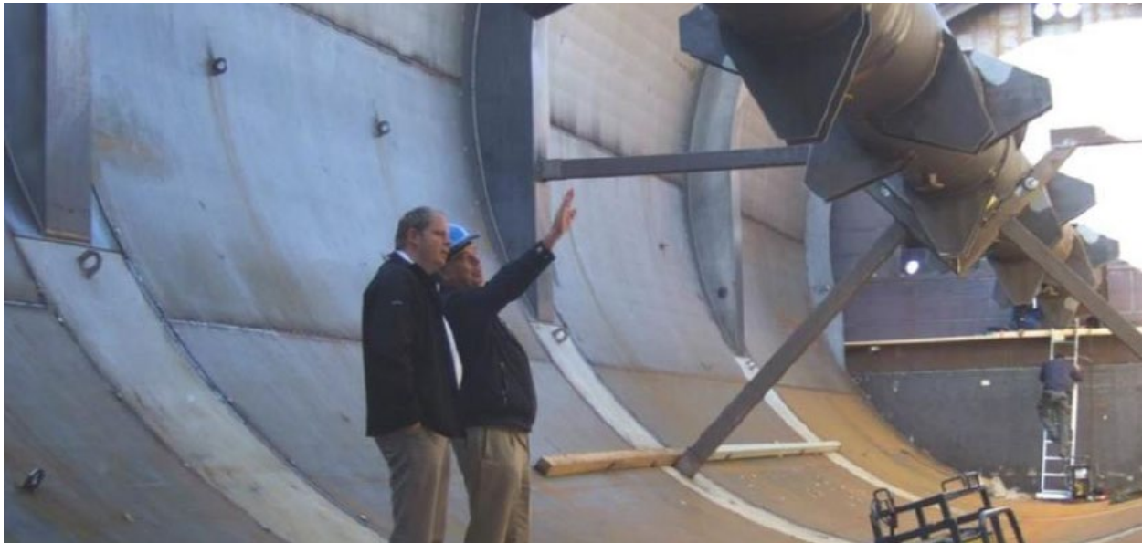
Figure 3-12. Interior of horizontal plug flow digester
