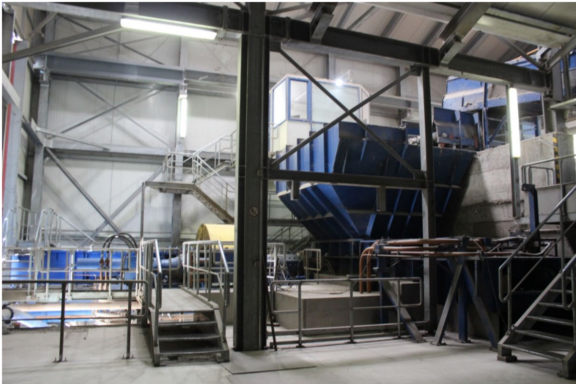
Figure 2-4. Anaergia, OREX, Kaiserslautern: feed hopper (right), OREX press (bottom left)
