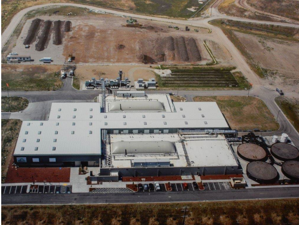
Figure 3-15. ZWED dry fermentation facility in San Jose, California (aerial view)
