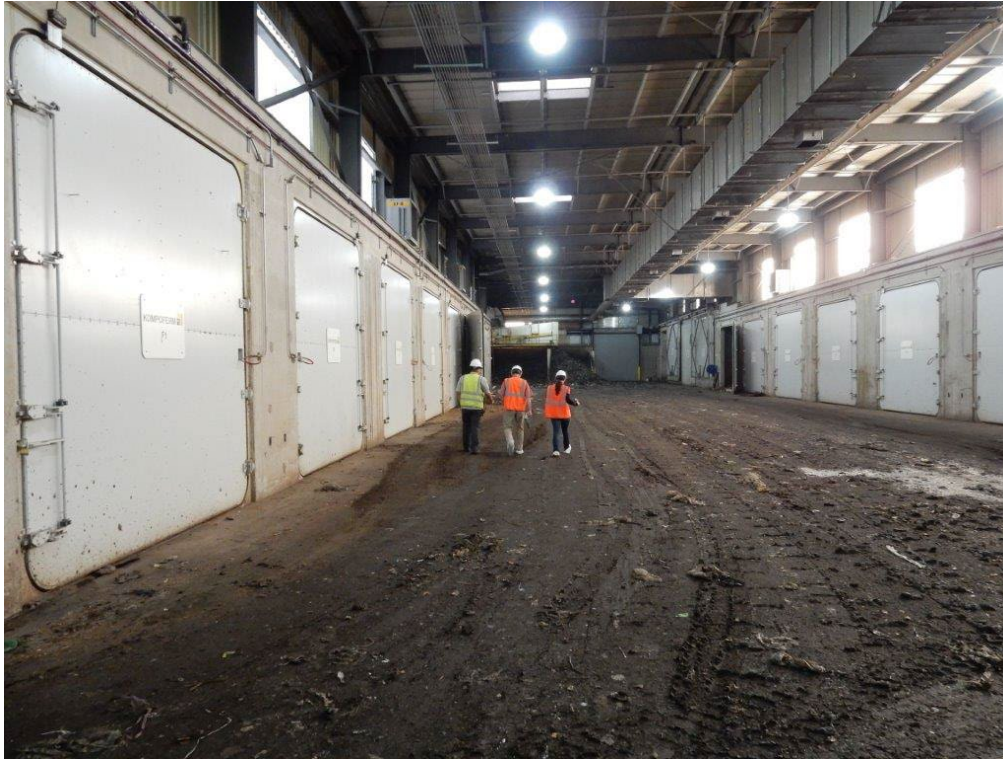
Figure 3-16. ZWED dry fermentation facility bunkers in San Jose, California (interior view)
