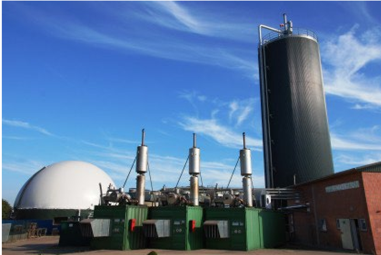
Figure 3-13. Vertical plug flow digester
