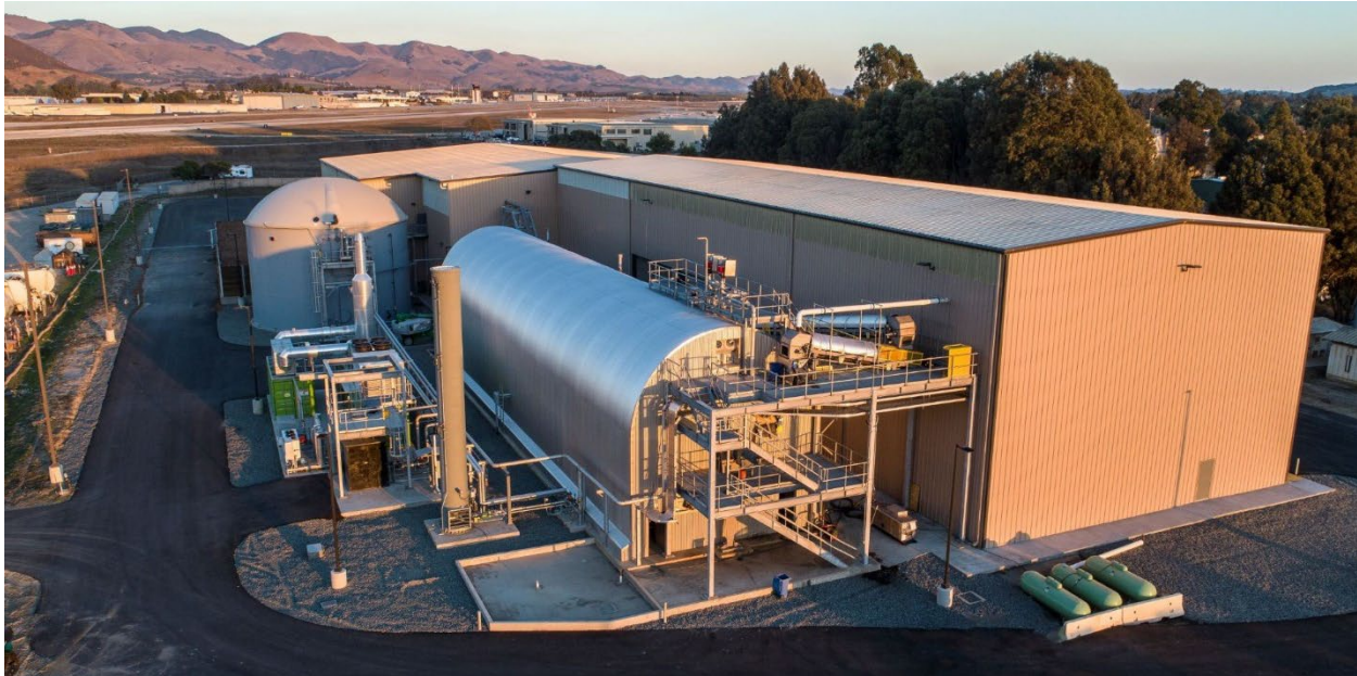
Figure 3-11. High-solids anaerobic digestion facility, San Luis Obispo, California
