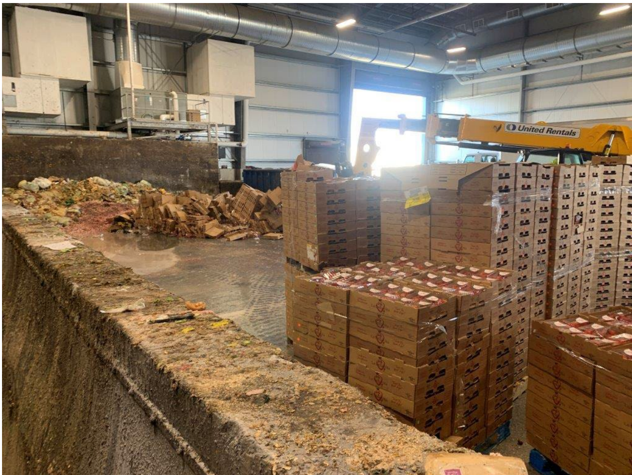
Figure 3-5. Receiving Building at Bioenergy Devco AD facility
