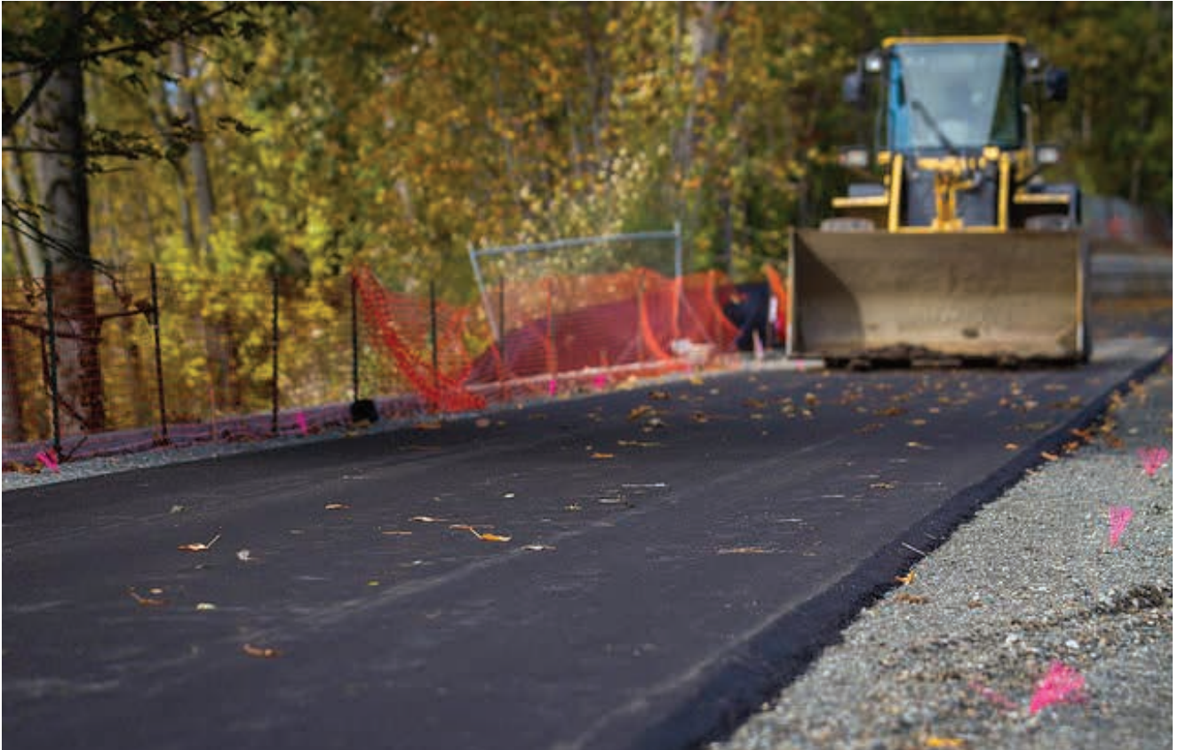
East Lake Sammamish Trail Construction
