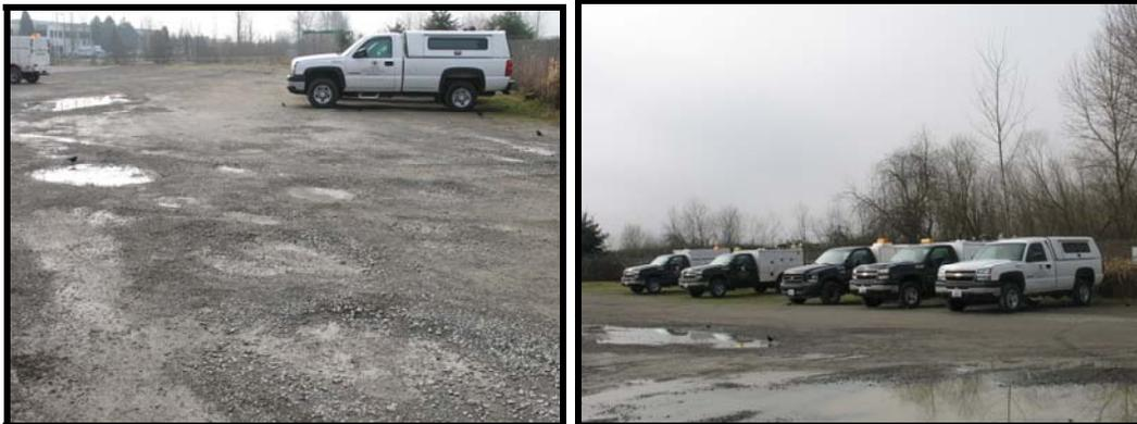
*Potholes flood during rainy weather, and provide for a very bumpy ride at the Kent facility, especially in the area where animal control transport vehicles are bringing animals into the facility. (Page 45)*
