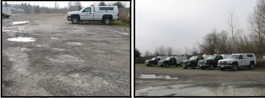
*Potholes flood during rainy weather, and provide for a very bumpy ride at the Kent facility, especially in the area where animal control transport vehicles are bringing animals into the facility.*
