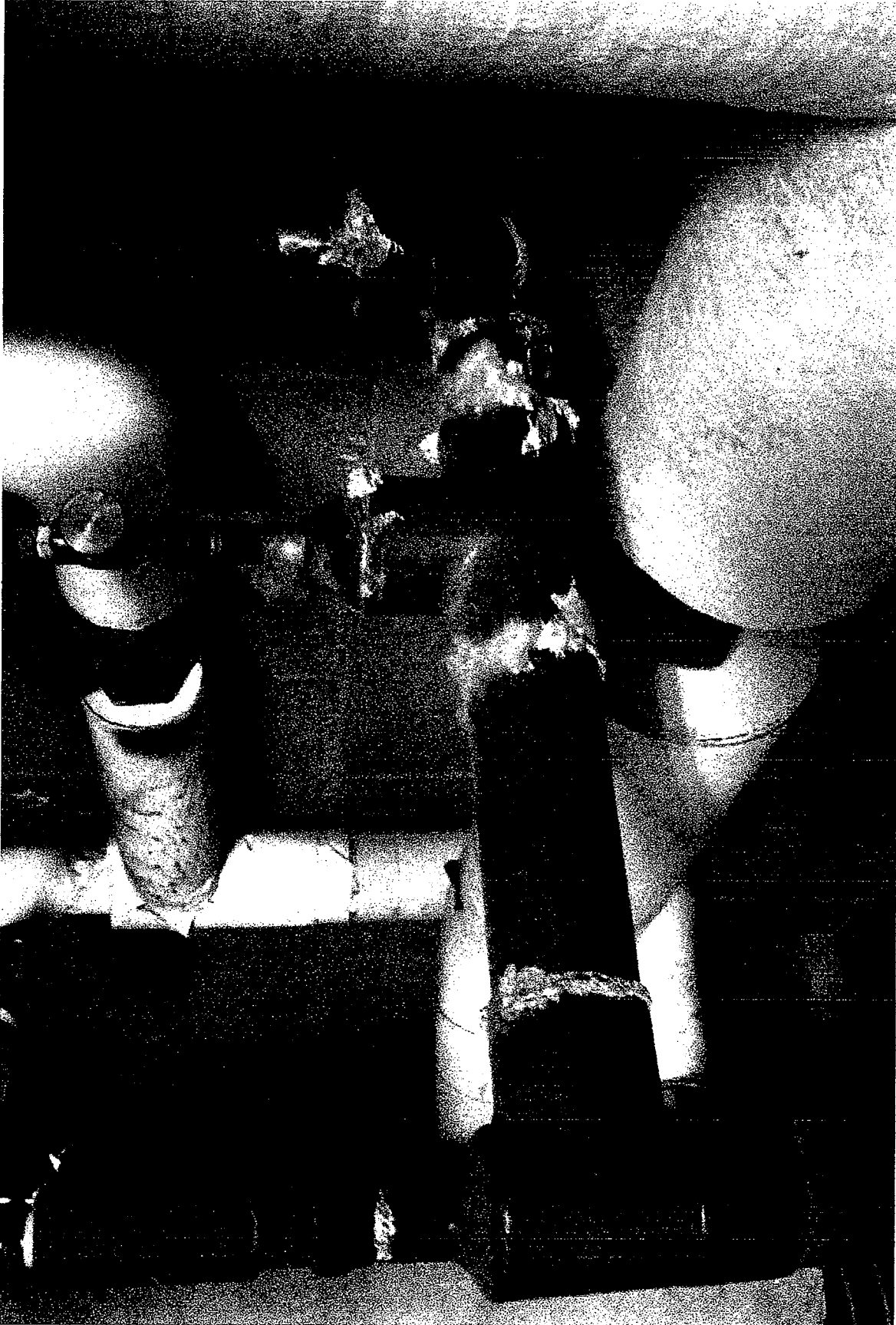
P-2 Pipe At Water Heater Crystalline substance is a salt-like structure. Fuzzy material is leftover fiberglass insulation.
