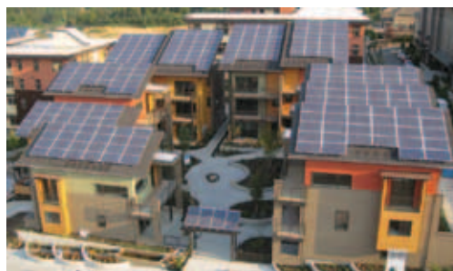
zHome zero-energy project in Issaquah
