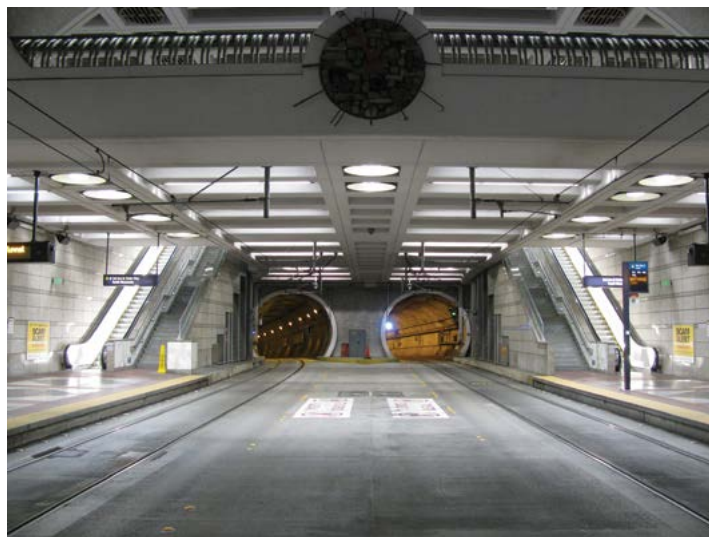
Over the past three years, Metro Transit has installed LED lights in the downtown Seattle transit tunnel that have reduced energy use by 21% compared to 2009, saving over $130,000 in energy costs per year.
