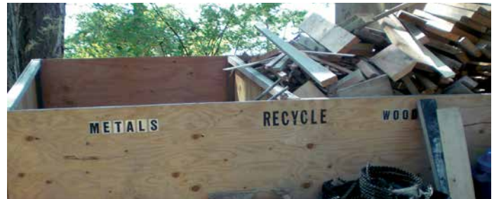
Separating waste onsite helps improve the overall recycling rate and can save you money.
