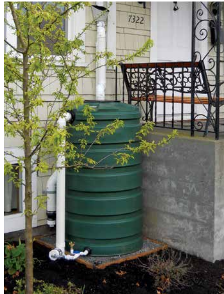
Rain barrels and cisterns provide an easy option for collecting rainwater to use within your landscaping. Source: King County .
