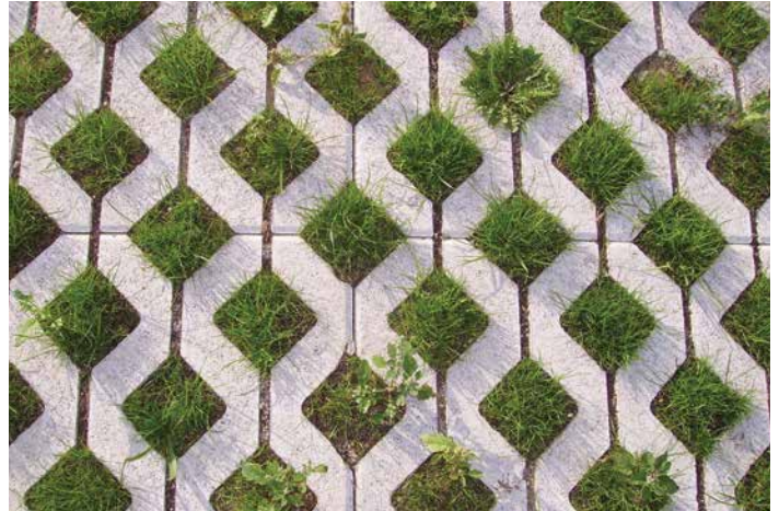
Permeable grass pavers are an attractive permeable alternative for parking areas and patios.
