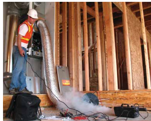
Duct leakage testing in a new home. Non-toxic smoke can be used to locate leakage areas, especially during framing in new construction. Source: O'Brien & Company.
