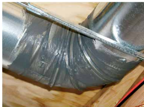
This metal duct elbow seam is properly sealed with duct mastic. If the ducts are in the crawl space, attic, or garage, they should be insulated after being well sealed. Source: O'Brien & Company.
