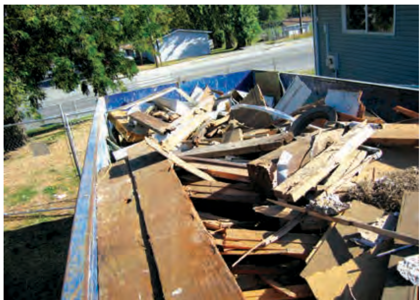
Container with construction and demolition debris for recycling
