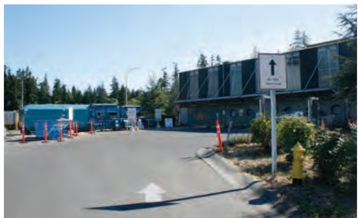
The Vashon Recycling and Transfer Station
