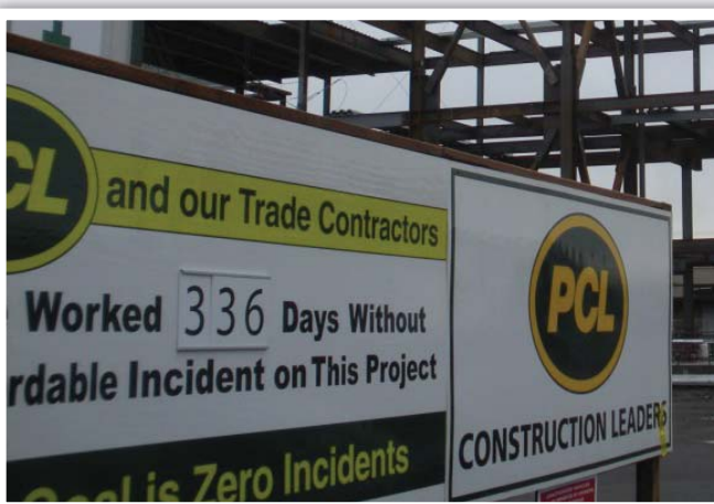
PCL jobsite signage for sharing safety achievements.
