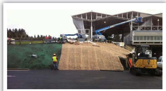
Houghton Transfer Station erosion control matting installation.
