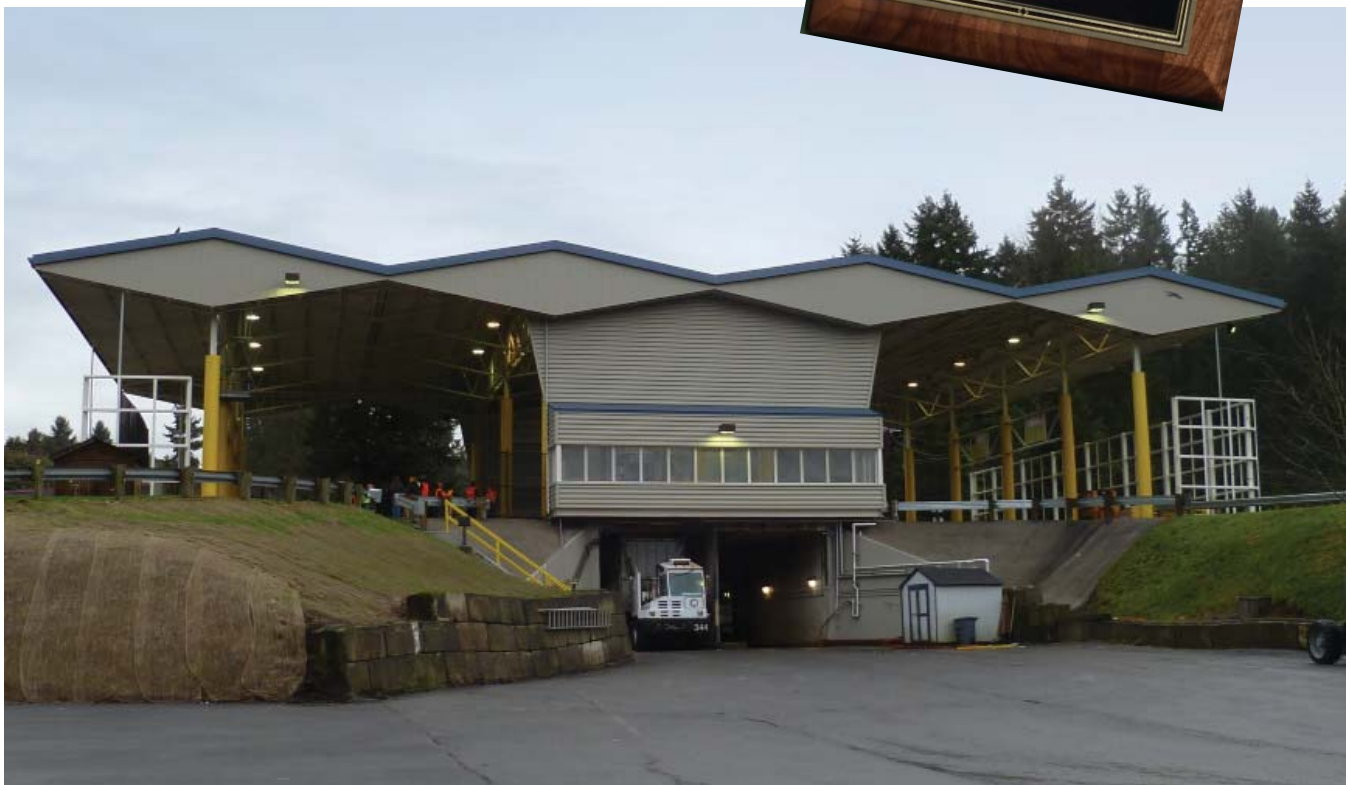
Houghton Transfer Station Roof Improvement and Mitigation Project
