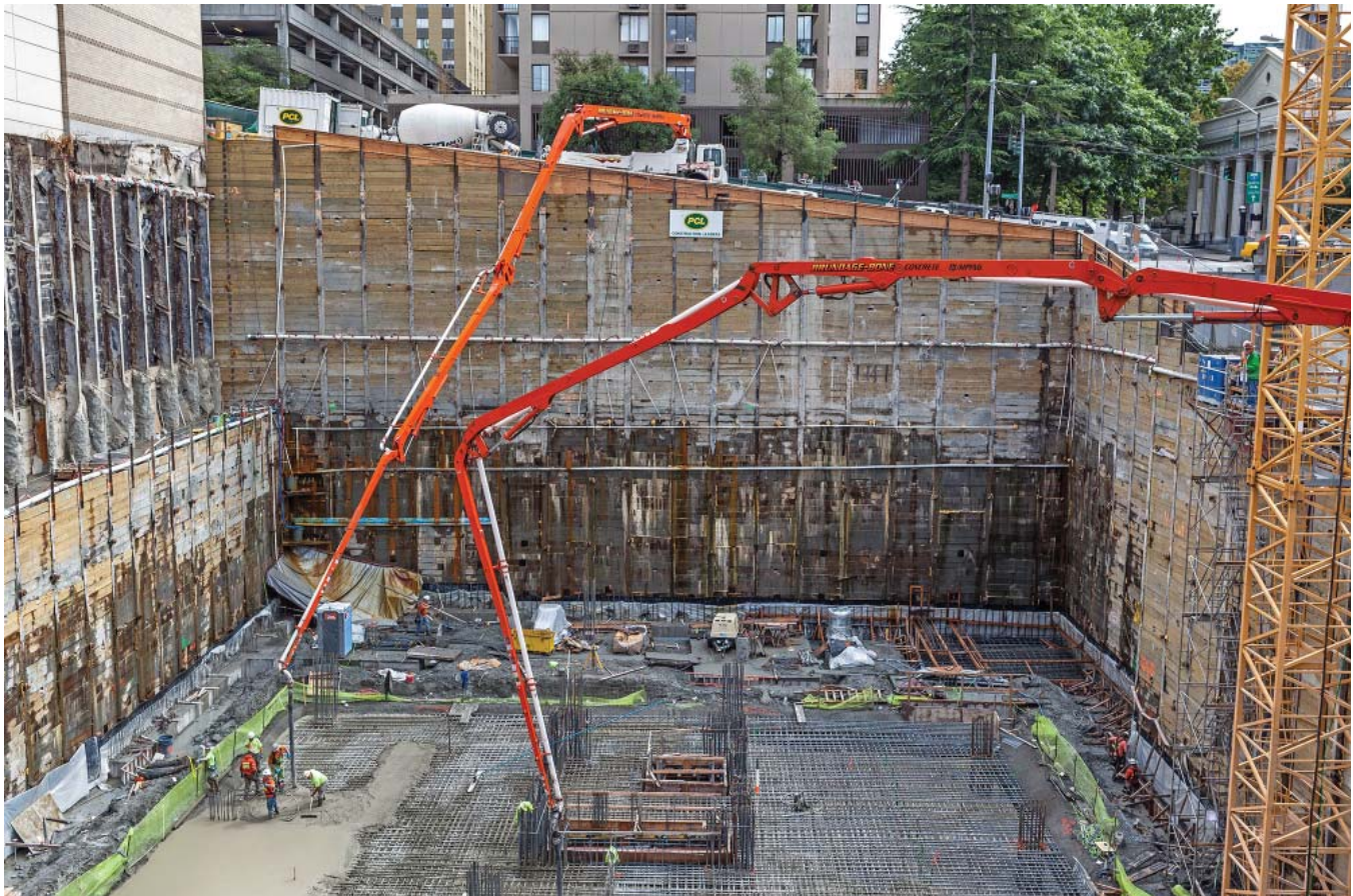
Seneca Apartment Community Concrete Pour August 29, 2013
